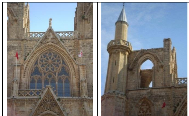
Figure 3.16. Famagusta, St. Nicholas Cathedral, c.14 th Century. Details of the Western Façade Window and the North-Western Bell Tower with the Minaret Added during the Ottoman Empire (©G. Pirlanta).
