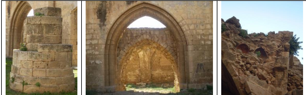
Figure 4.36. Famagusta, St. George the Greek, c.14 th Century. i. Piers of the Nave. ii. Gothic Arches of St. George and St. Simeon Churches. iii. Potteries Inserted into the Apse Vault (©G. Pirlanta).
