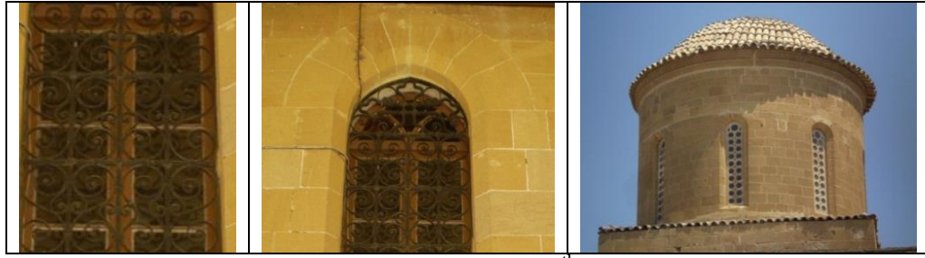
Figure 4.22. Morphou, St. Mamas Church, c.18 th Century. Window Grills with Hellenistic Motif, 20 th century and Byzantine Round Arch and Dome, c. 18 th century (©G. Pirlanta).
