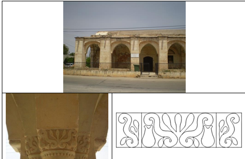
Figure 4.68. Limnia, St. George Church, c.19 th Century. i. Portico Built with Ashlar Blocks of Limestone. ii.- iii. Hellenistic Style Capitals in the Portico (©G. Pırlanta).
