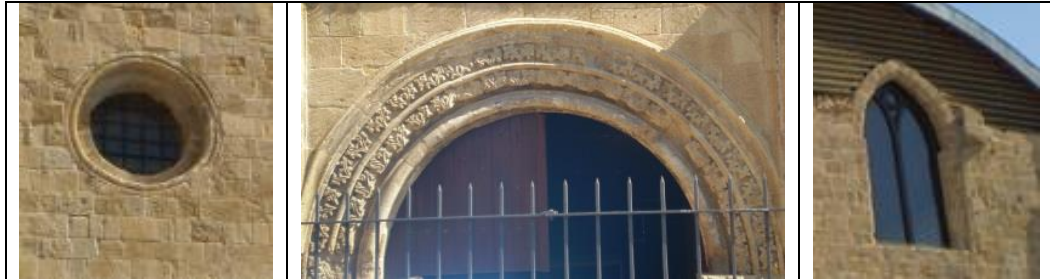
Figure 4.5. Nicosia, St. Nicholas Church, c.5 th Century. Byzantine Style Rose Window and Round Arch and Gothic Style Openings on the West and Eastern Façades (©G. Pirlanta).
