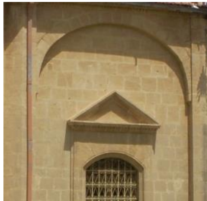
Figure 4.61. Kythrea, St. George Church, c.19 th Century. Hellenistic Style Pediment Over the East Window Pediment (©G. Pirlanta).
