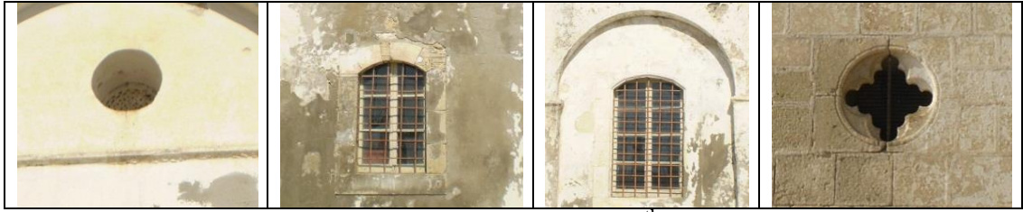
Figure 4.39. Rizo Karpaso, St. Synesios Church c.18 th Century. Different Styles of Windows (©G. Pirlanta).
