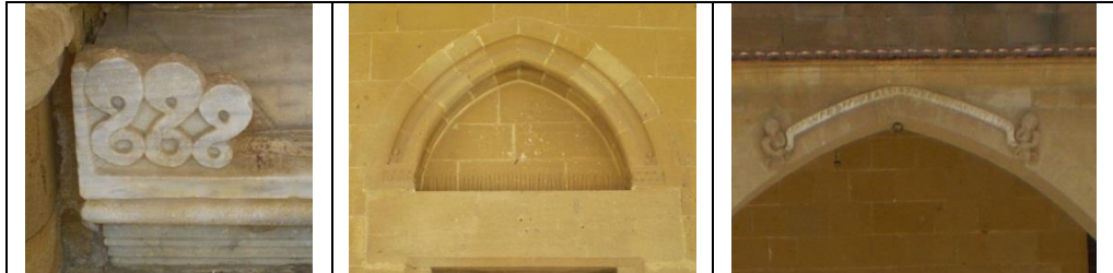
Figure 4.21. Morphou, St. Mamas Church, c.18 th Century. Tomb of Saint Mamas, Portal Ornamentation with Rosette Motif in Hellenistic Style and Gothic Style Tympanum and Inscription Banner on the Northern Façade (©G. Pirlanta).
