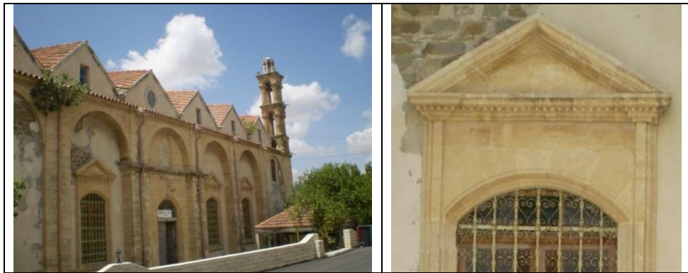
Figure 4.60. Kythrea, St. George Church, c.19 th Century. Hellenistic Pediments on the Northern Façade (©G. Pirlanta).
