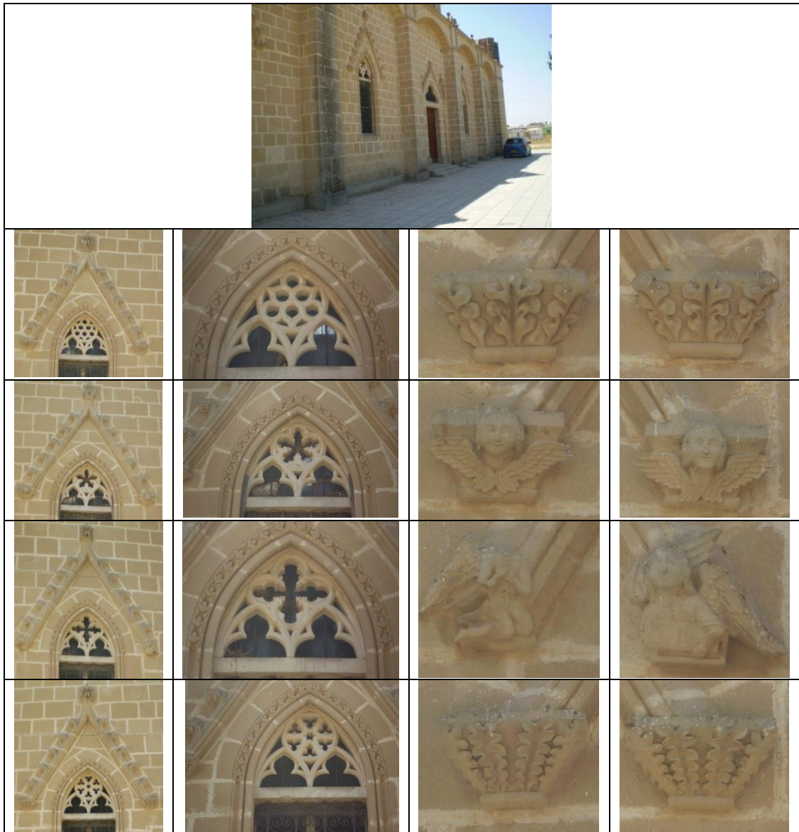
Figure 4.50. Lysi, Blessed Virgin Mary Church, 1880-1908. Window Characteristic of North Façade in Hellenistic, Byzantine and Gothic Styles (©G. Pirlanta).
