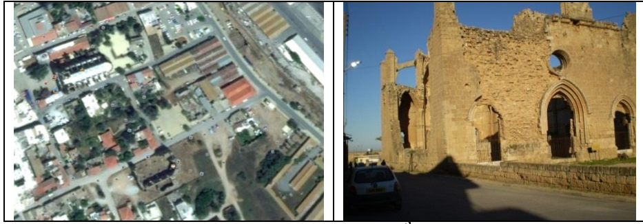
Figure 4.31. Famagusta, St. George the Greek, c.14 th Century. Site Plan and Western Façade of the Church (©G. Pirlanta).
