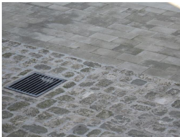
Figure 60: Pavement on the square
