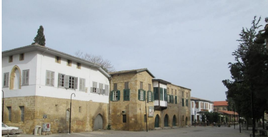
Figure 42: Restored traditional façade
