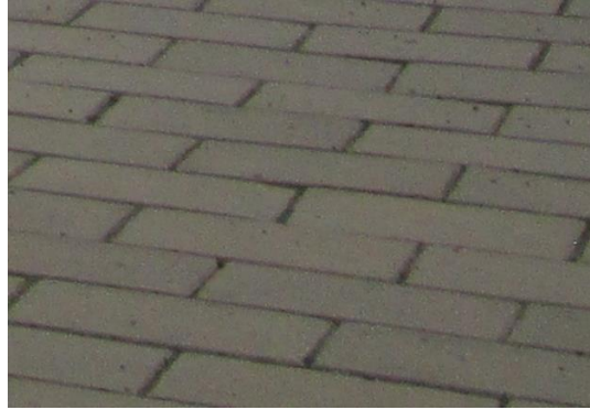
Figure 46: Pavement on the square
