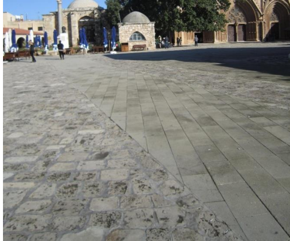
Figure 61: Pavement with mix materials
