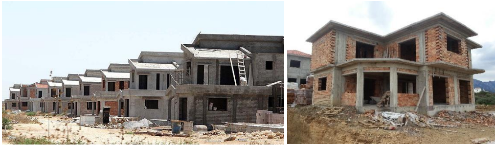
Figure 39 and 40. Construction in North Cyprus (URL 2, 3)
