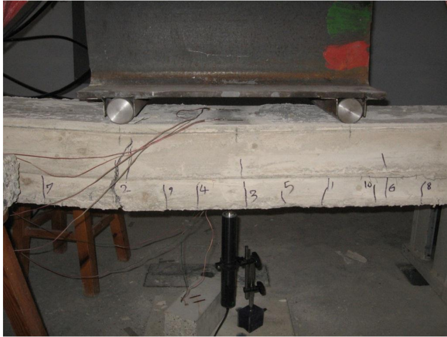
Figure 39: Crack pattern for concrete C40 (2%SP-0%Fiber)
