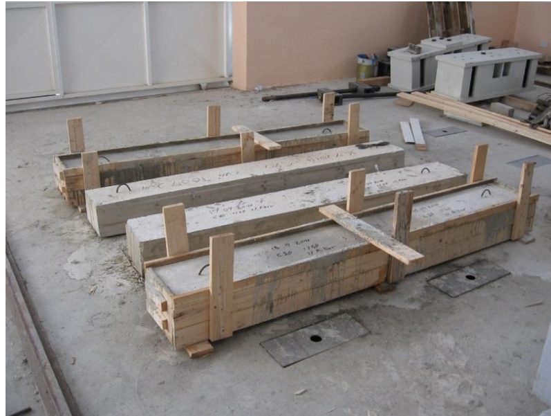
Figure 34: Slab filled with SCC
