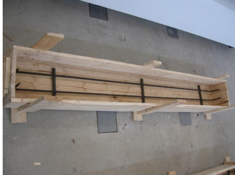
Figure 33: Slab formwork and steel bars
