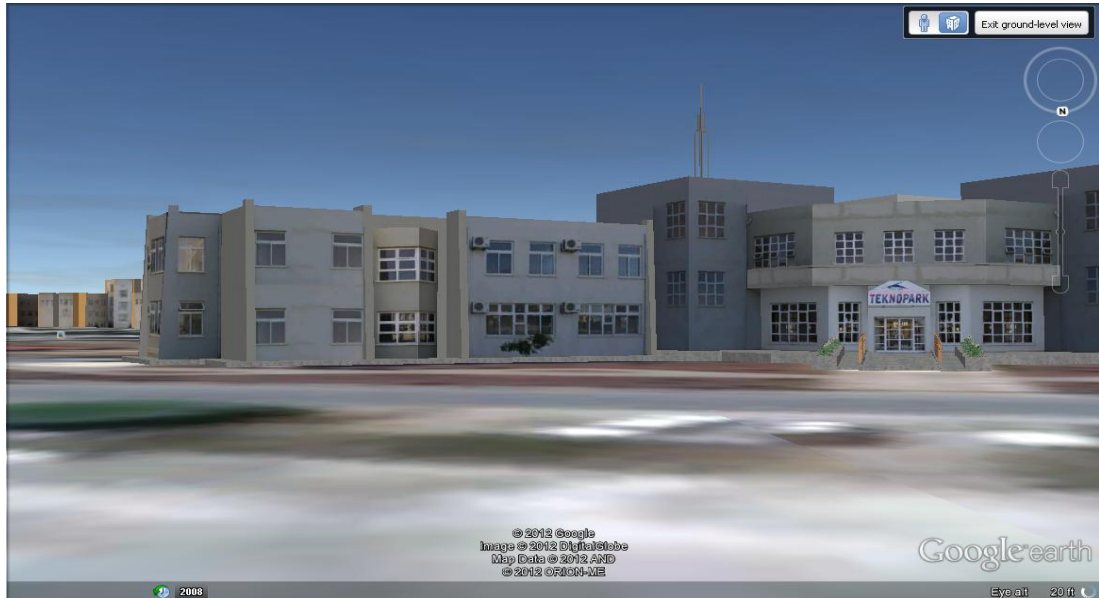
Figure 54: A 3D view of the western side of the entrance gate
