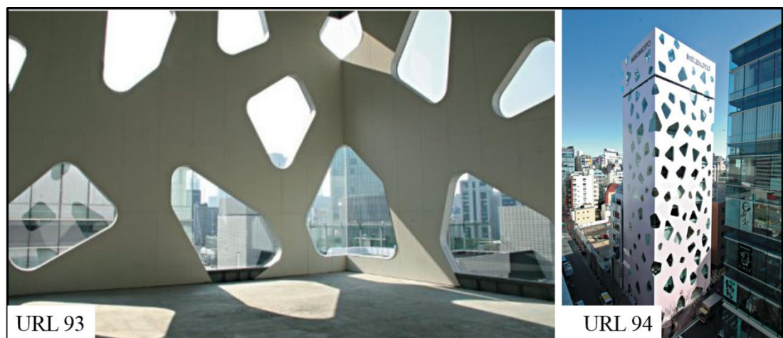
Figure 58: Different shapes of openings makes different effect on the light coming in and creates subspaces.
