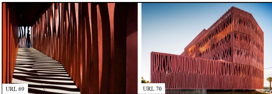
Figure 42: International Accommodation Center for the Oenological Observatory designed by Atelier Fernandez & Serres
