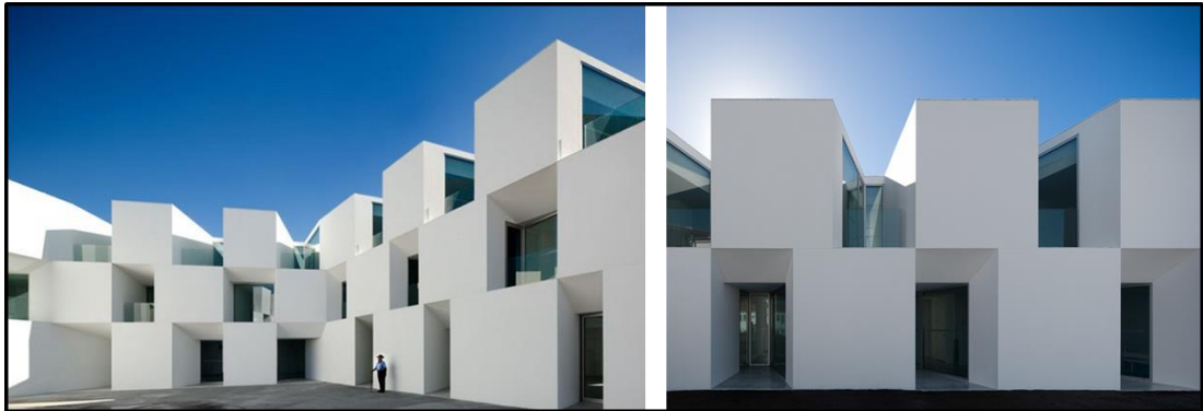
Figure 45: Volumetric elements create opening in Alcaces do Sal Residence designed by Aires Mateus URL 74)
