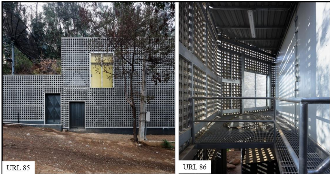
Figure 54: Texture created by natural lighting in the space - Transmission Central / UMWELT + Juan Manuel Sepúlveda
