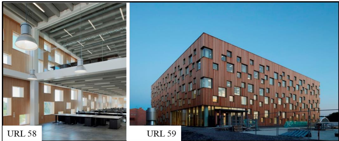
Figure 37: Variety in the size of openings in the Umea school of architecture
