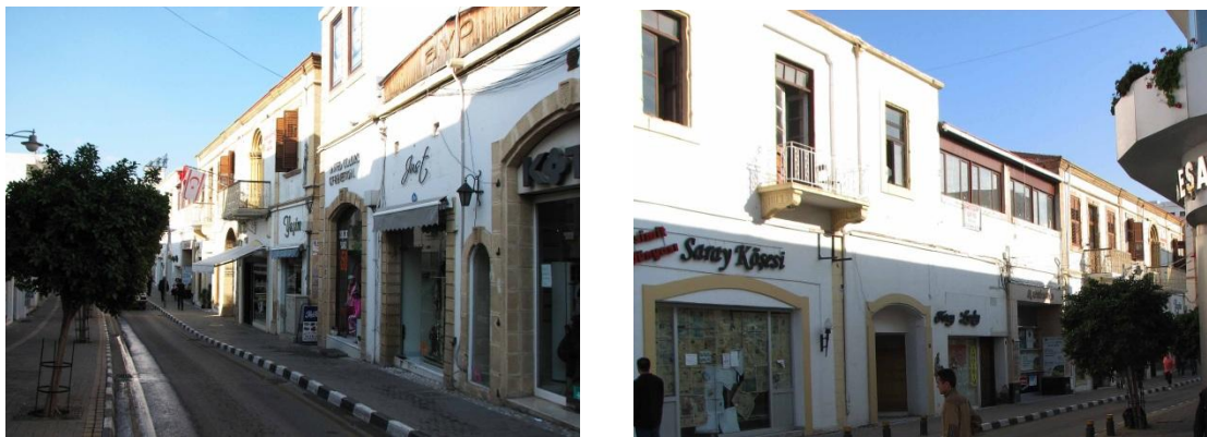
Figure 64: The historic buildings with similar heights and materials along the street (source: author)
