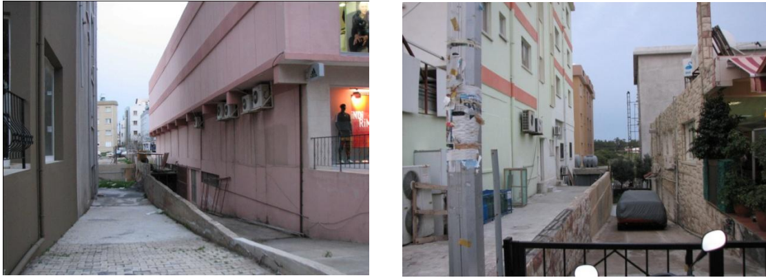
Figure 26: The gaps between each two building make an undesirable image of urban form (source: author)
