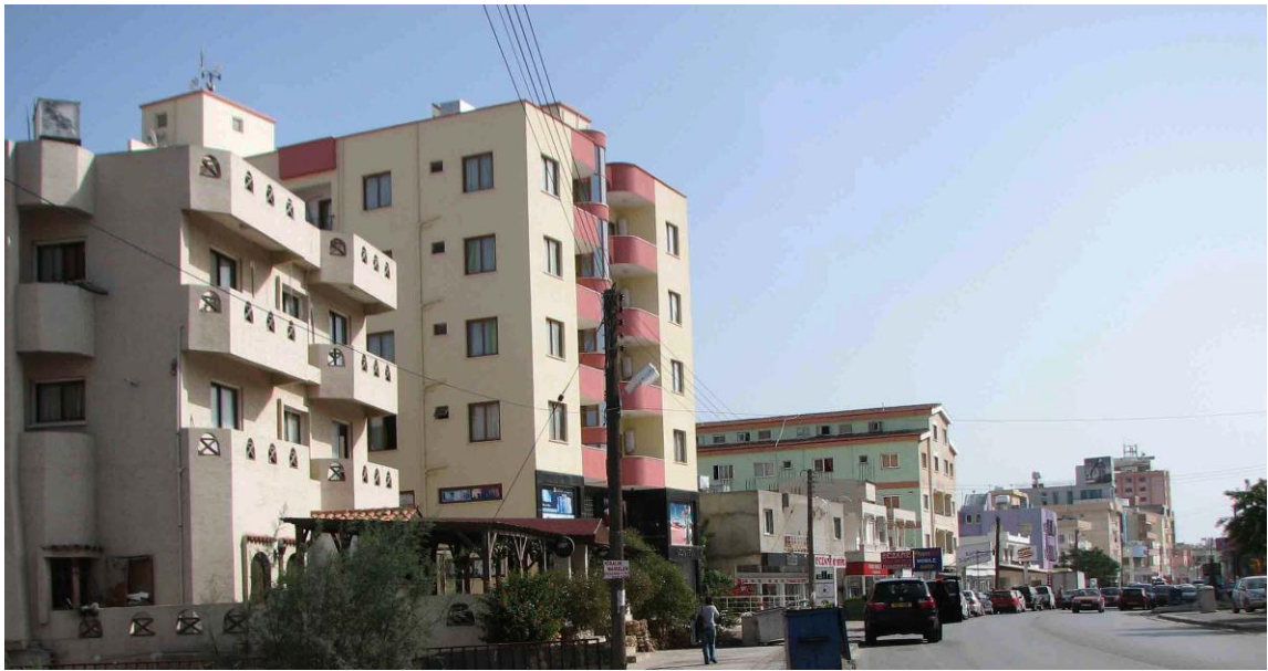
Figure 25: Chaos in view of the street which made of inharmonious buildings (source: author)
