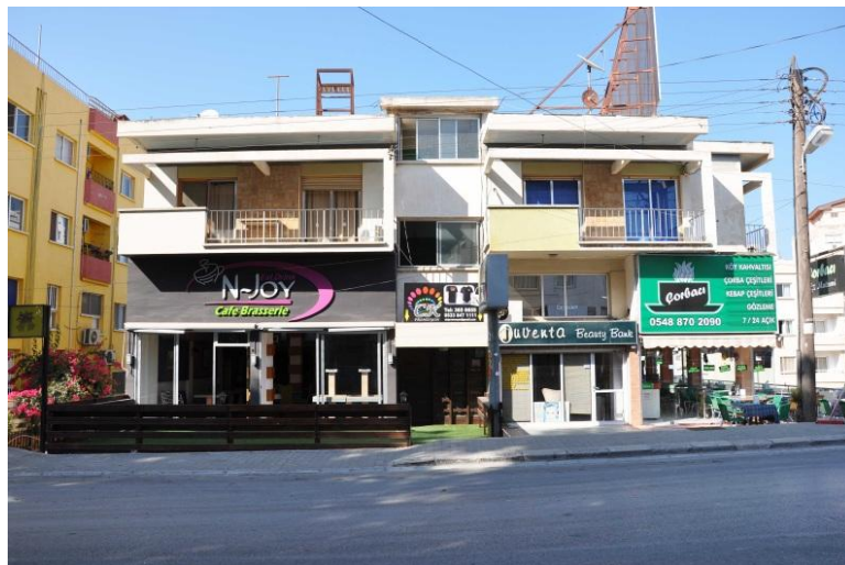
Figure 30: Multi-functional buildings are parts of the character of Salamis Street (source: author)
