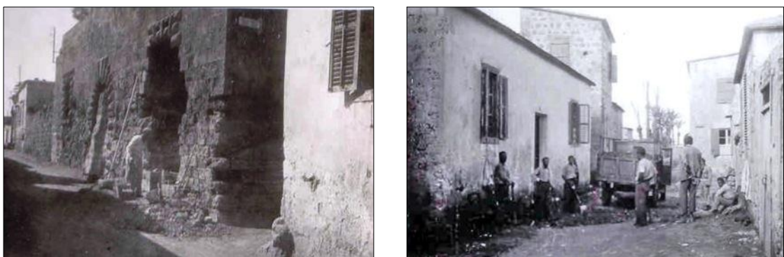
Figure 3.13. Digging process 1964 (National Geographic, 1964)
