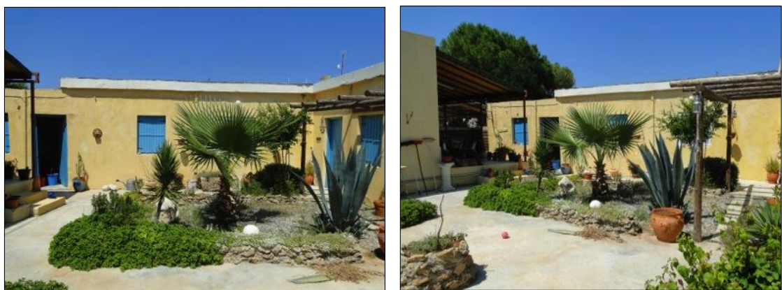
Figure 3.36. The courtyard after renewal (Author, 2012)
