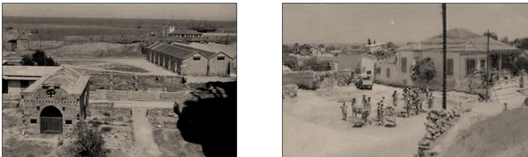
Figure3.6. The storage buildings and a British house (National Geographic, 1957)
