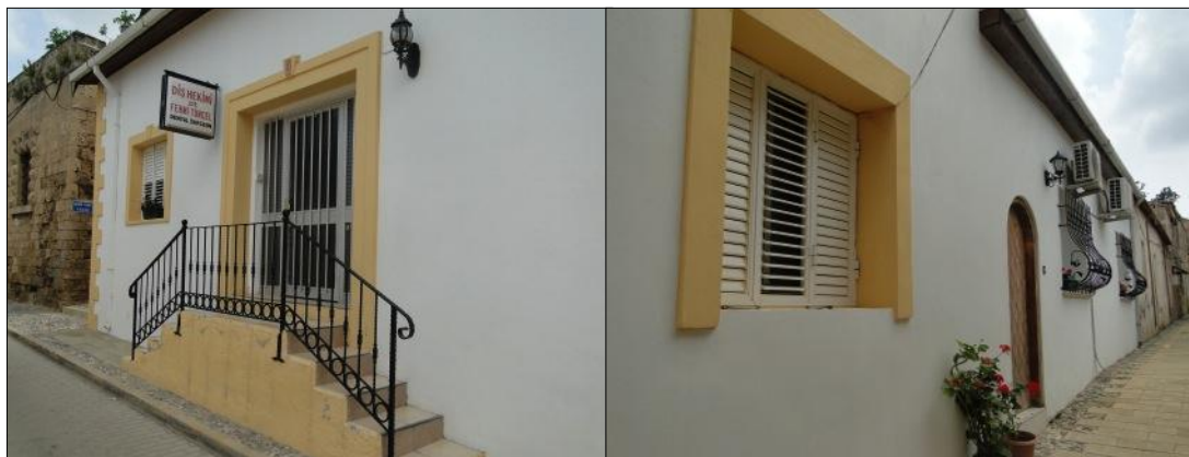
Figure3.11 The entrances of the house (Author, 2012)
