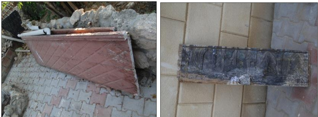
Figure3.4 5. The original door of the entrance and windows frame (Author, 2012)
