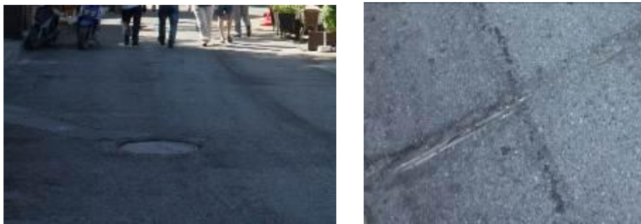
Figure 4.20: Wheels Getting Caught in the Grates
