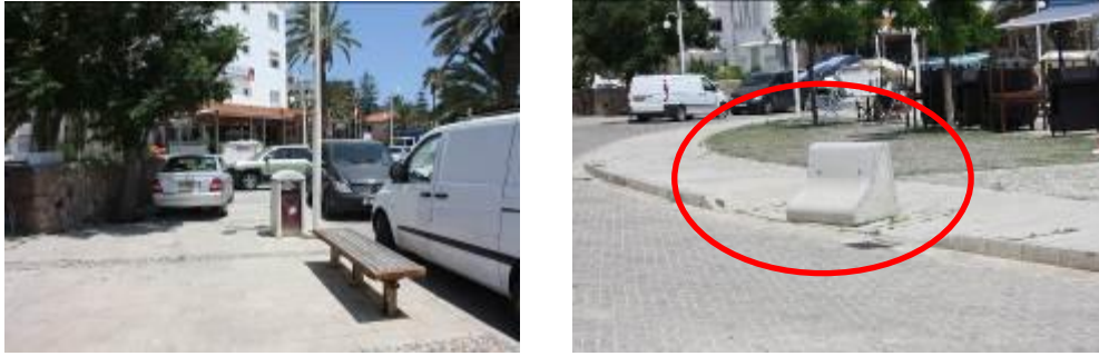
Figure 4.61: Decreasing the Width of Curb Ramp with Cars & Barriers As Obstacles
