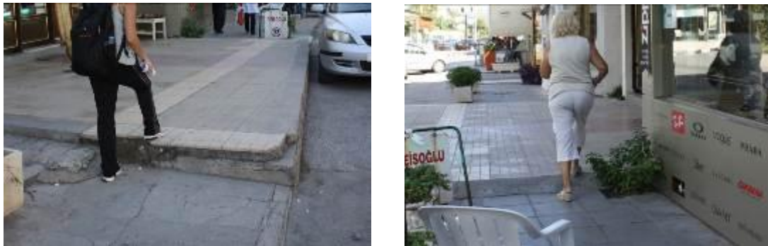
Figure 4.45: Lack of Ramp Provide Problem and Limitation for the Disabled
