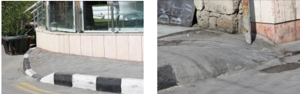
Figure 4.44: Inappropriate and Hazardous Curb Ramp.
