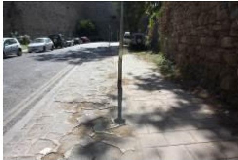
Figure 4.9: Due to Lack of Furniture, Lighting and Signs Cause Unfamiliar and Unsafely Environments.
