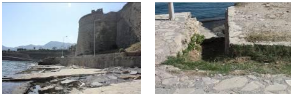
Figure 4.14: Poor Maintenance of the Material Covering.
