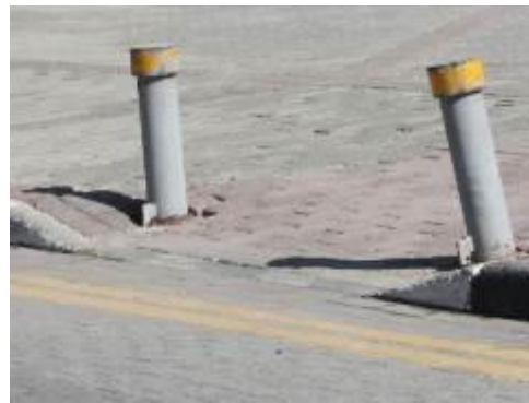
Figure 4.36: Obstacles Create Inaccessible Curb Ramp
