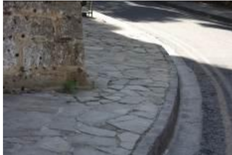
Figure 4.5: Lack of Curb Ramp and Inappropriate Width Cause Limitation for Travelling in the Street
