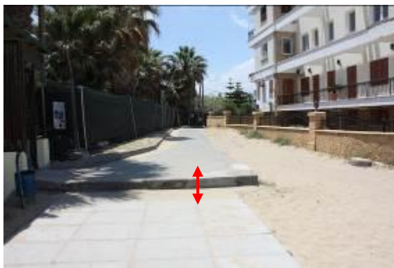
Figure 4.71: Lack of Curb Ramp
