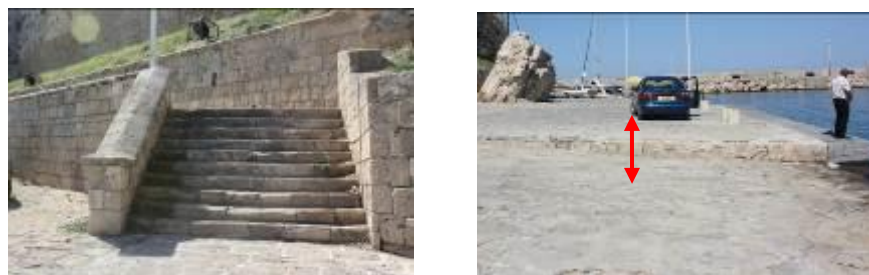
Figure 4.15: Lack of Ramp and Beveled Edge Create Problem for Wheelchair Users.
