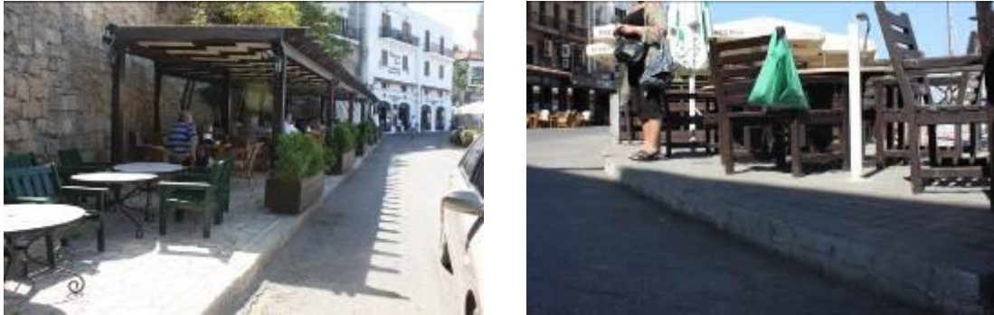
Figure 4.21: Change in Level Needs Ramps or Curb Ramps to Improve Accessibility.
