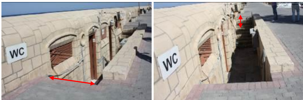
Figure 4.25: Inaccessible Services (WC.).
