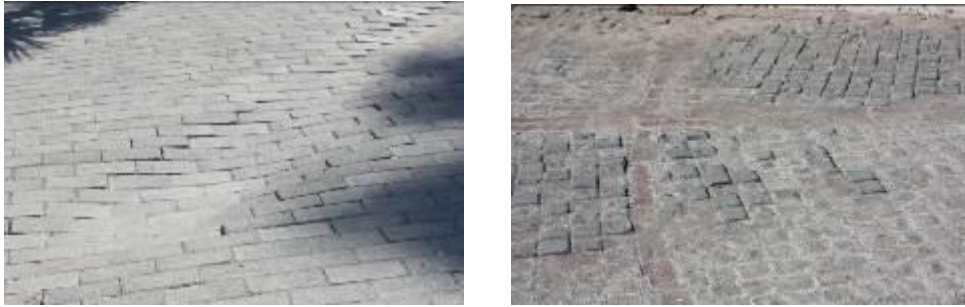
Figure 4.34: Poor Maintenance Can Restrict Access & Threaten Safety for the Disable.
