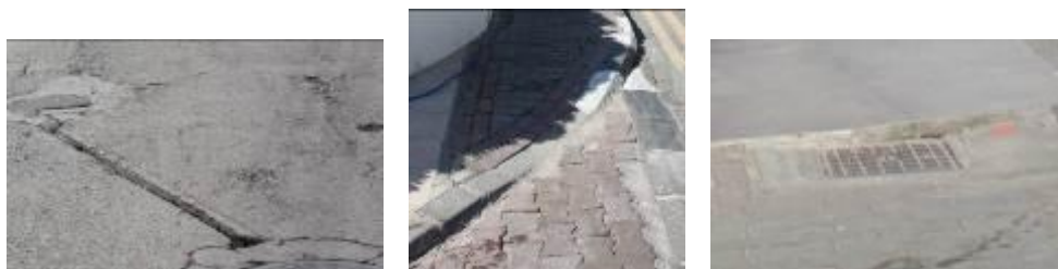
Figure 4.43: Gaps and Opening Create Problem at Street 8.
