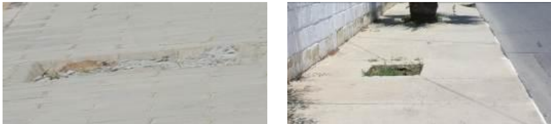
Figure 4.64: Gaps and Grates Create Dangerous for Disables.
