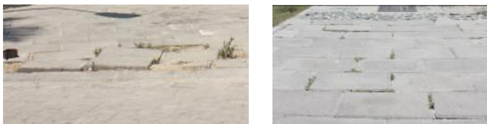
Figure 4.65: Lack of Maintenance Cause Danger for Everybody.
