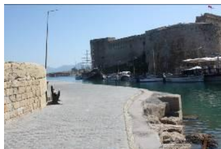
Figure 4.30: Lack of Edge Protection Causes Unsafe Space.
