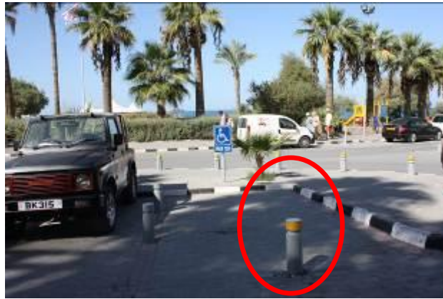
Figure 4.52: The Parking Space Is Not Only Obstructed with Obstacle, But Also There Is Not Any Curb Ramp.
