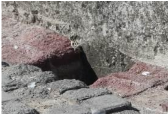
Figure 4.35: Drainage Cause Control Lose & Create Tripping Hazard.
