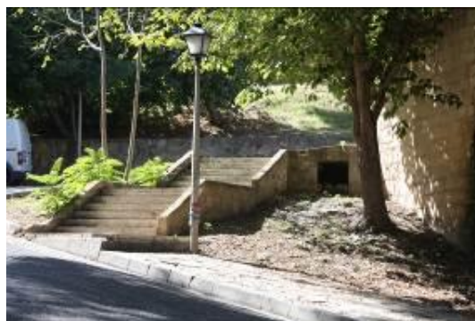
Figure 4.8: Inaccessible Stair Box.
