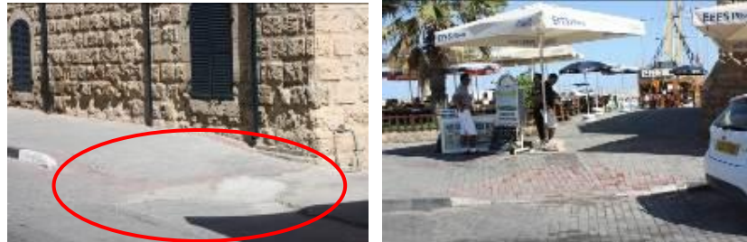
Figure 4.28: Available Curb Ramps in Zone 1 at Street 6.
