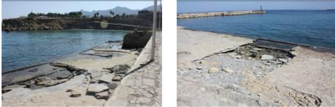
Figure 4.13: Tripping Hazard and Deep Gaps.
