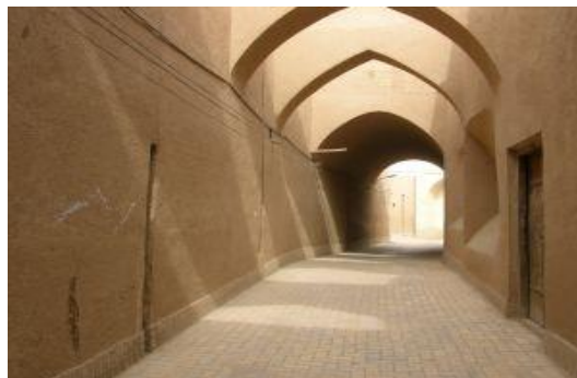
Figure 2.5: A Narrow and Enclosed Street in Yazd Because of the Weather. This Form Creates Shading in Very Hot Climate. (URL 3)
