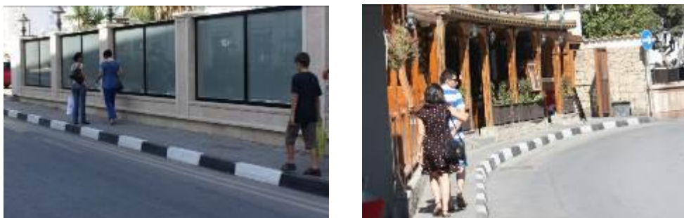
Figure 4.41: Lack of Sidewalk and Unsuitable width for Sidewalk Creates Risk for the Disable.
