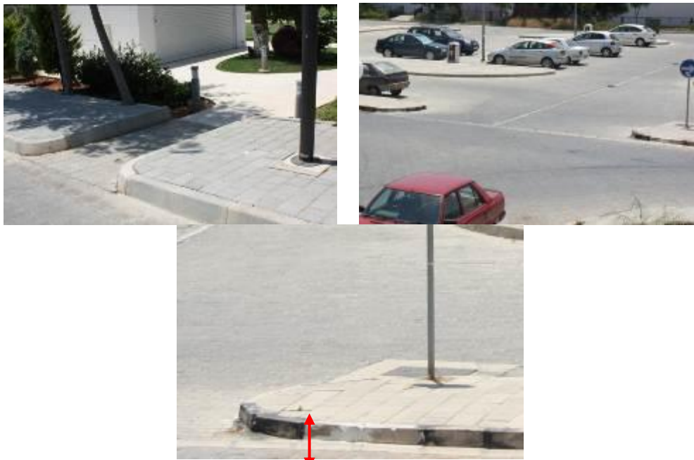
Figure 4.66: Lack of Ramp in Vertical Displacements Limit the Disable
