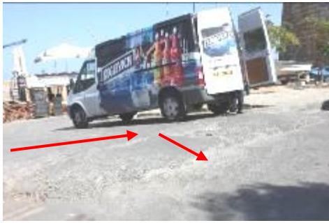
Figure 4.18: Because Two Different Slopes Arrive together without Landing the Path Create Problem.
