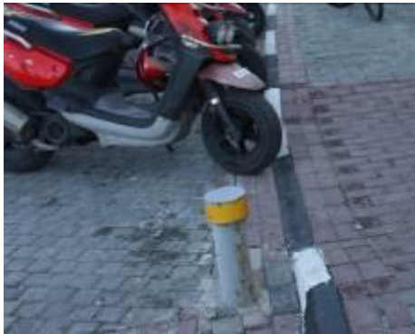
Figure 4.36: Obstacles Create Inaccessible Curb Ramp
