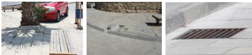
Figure 4.57: Lack of Maintenance & Dangerous Opening
