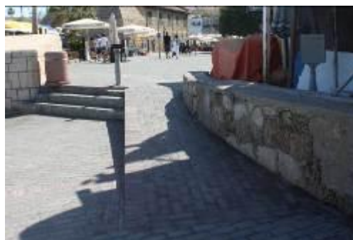
Figure 4.37: Non-Standard Stairs and Ramp According to Accessible Design.
