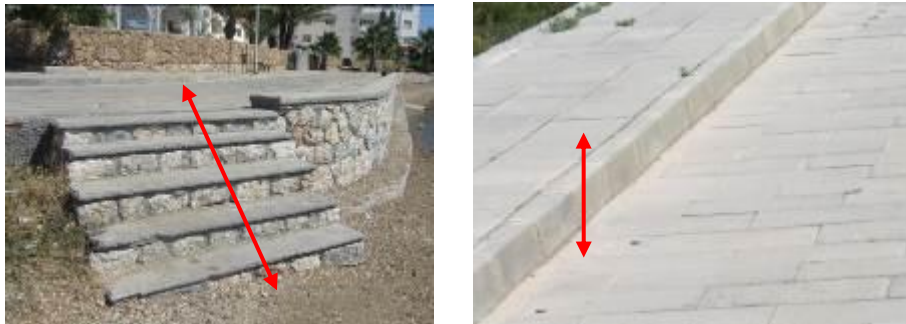
Figure 4.58: Lack of Ramp and Curb Ram.
