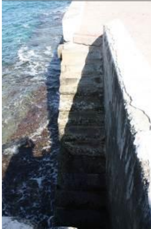
Figure 4.38: Dangerous Stairs at K.S.F.
