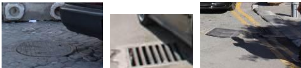
Figure 4.53: Gaps and Opening Provide Hazard for the Disabled.
