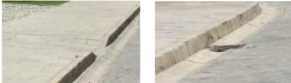
Figure 4.63: Dangerous Curb Ramp & Drain Channel.
