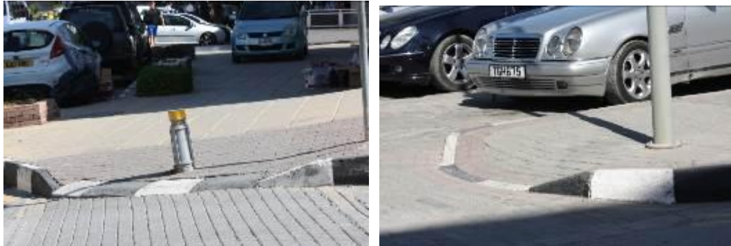
Figure 4.40: Dangerous and Terrible Design in Driveway Crossing.
