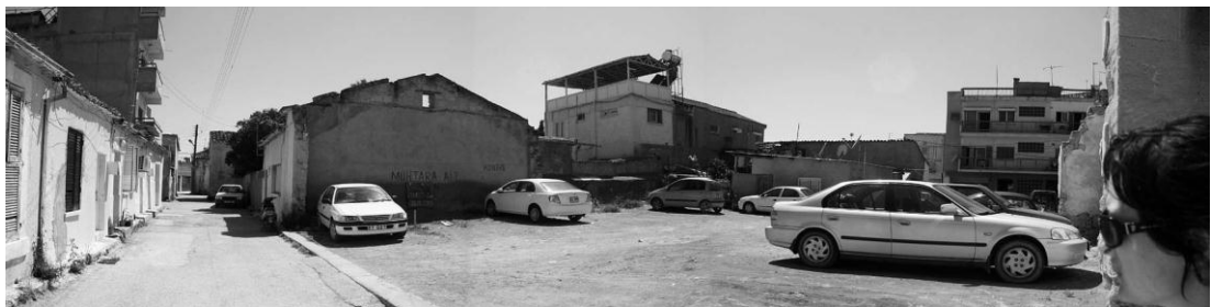
Figure 39. Vacant Lands are being used as a parking lot, Lack of permeability on the facades, by Author, 2012
