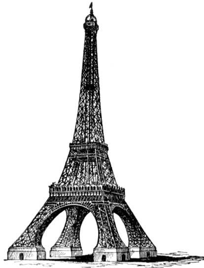
Figure 3.8: Eiffel tower, one of the first steel structures
