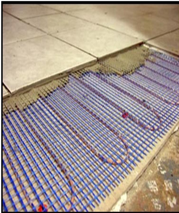
Figure 11: Radiant Underfloor Heating System ( http://www.ideal-heating.com/ )
