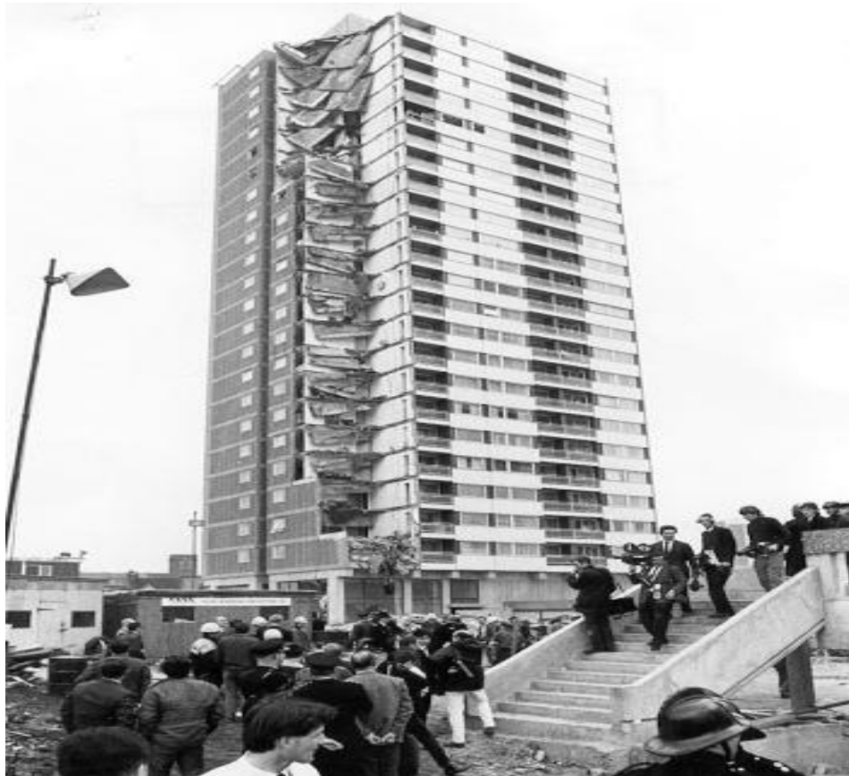
Figure 1: A partial collapse of the Ronan Point Apartment tower in 1968 (Wikipedia, 2012)
