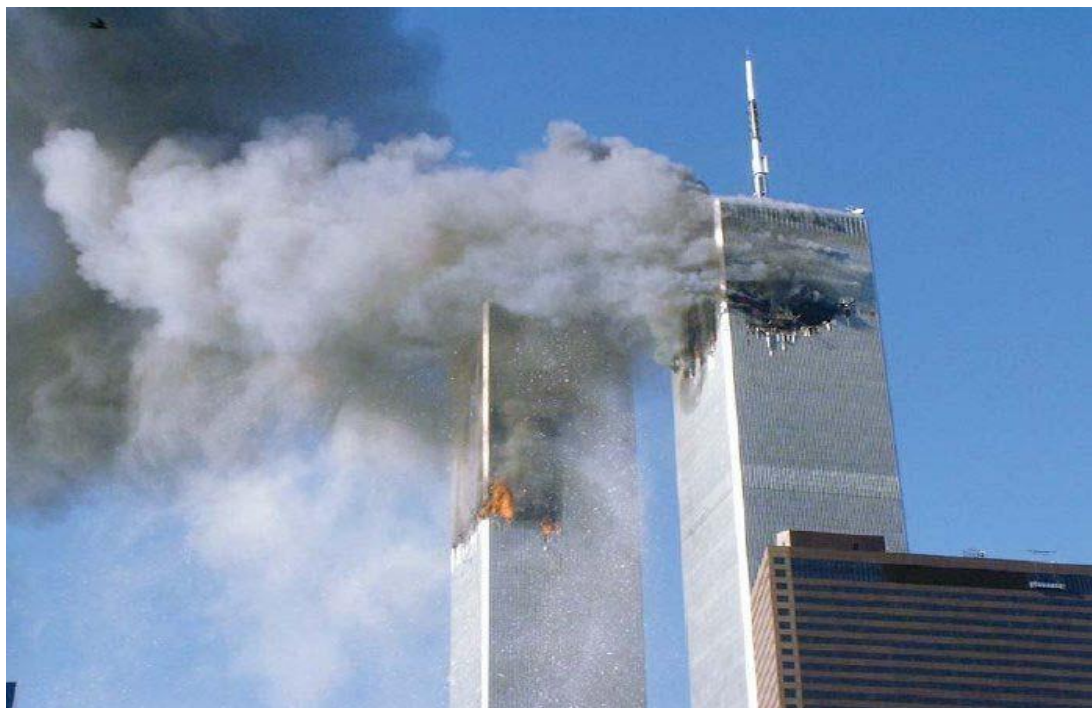
Figure 3: The north and east faces of the World Trade Center towers, showing fire and crash destruction to both towers (FEMA-403, 2002)
