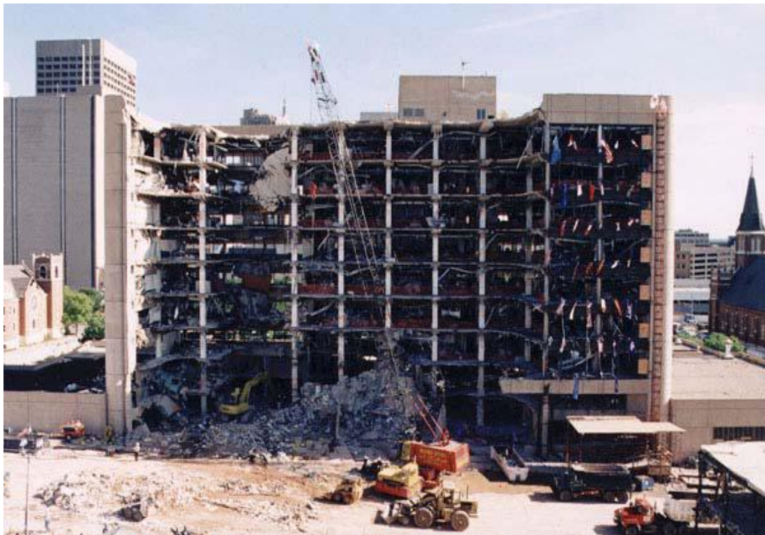
Figure 2: External sight of Alfred P. Murrah Federal building collapse (FEMA-427, 2003)
