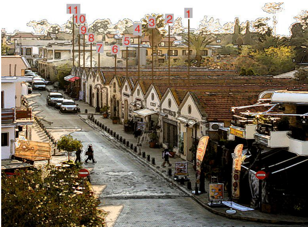
Figure 4.2: Warehouses in Liman road, the walled city, Famagusta
