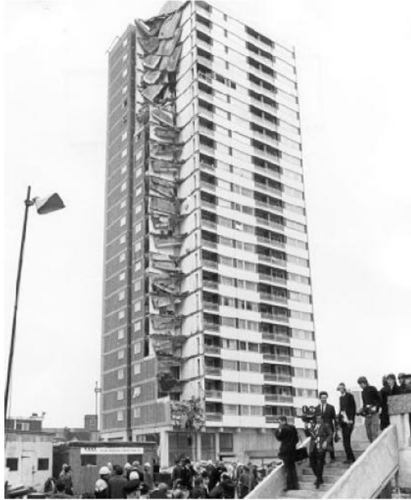
Figure 3: Progressive collapse in Ronan Point Building (16May 1968)
