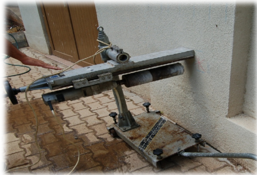
Figure 3-2 Obtaining cylinder concrete core sample from column
