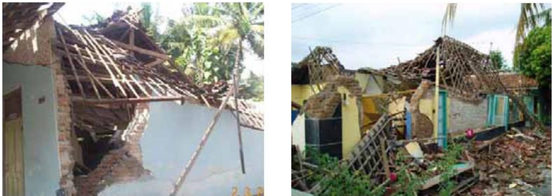
Figure 3-12: The destroyed masonry thick walled (old culture) (Boen, 2006)
