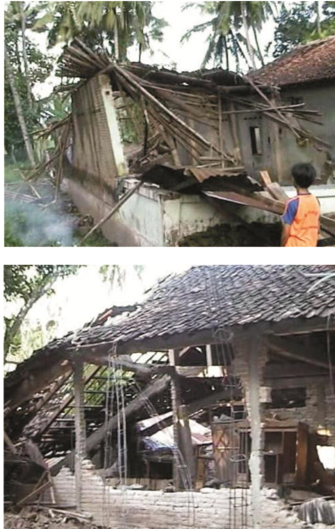
Figure 3-6: Sample of Destroyed houses from the 2006 earthquake; pure traditional, old culture, and new culture (Idham, N., et.al , 2010b)
