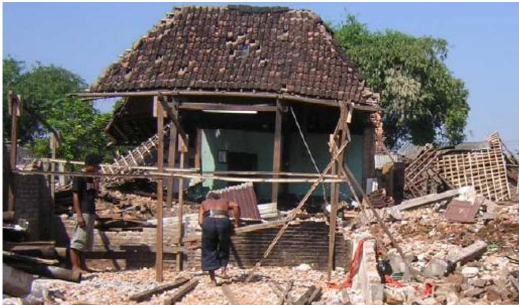
Figure 3-44. Destroyed traditional masonry house with remain four wooden columns standing (photo: BAPPENAS, 2006b)
