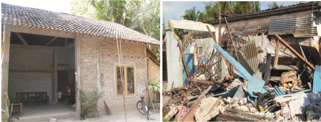
Figure 3-37: Wide opening house and the result sample after earthquake
