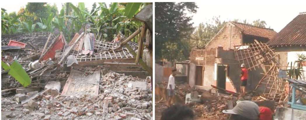
Figure 3-36: The result of thin and weak masonry wall usage after earthquake
