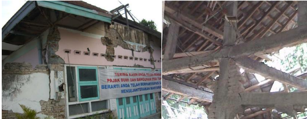
Figure 3-28: Damages on modern-vernacular type of the houses constructed by masonry and RC frame
