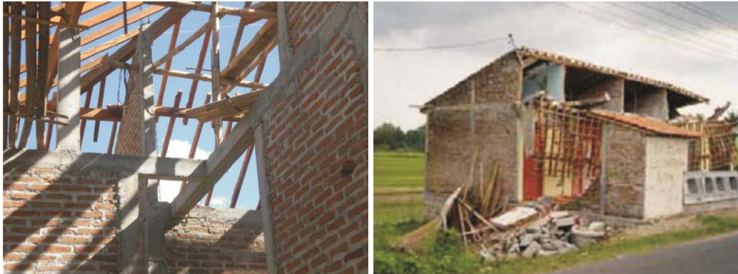
Figure 3-42: Complicated roof frame and result the failure after earthquake (right photo: Boen, 2007)
