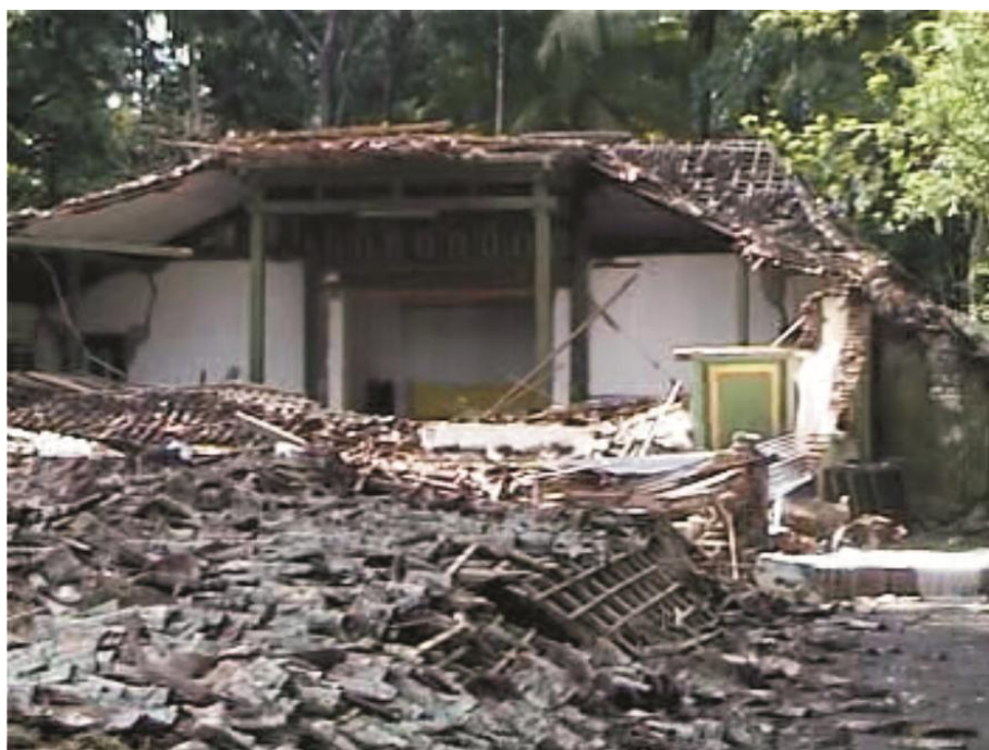
Figure 3-27: The remain standing four main columns Saka Guru
