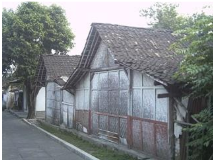
Figure 3-2 Original Javanese Joglo , Limasan , and Kampung types with clay roof tiles and wooden materials ranging from hardwood to bamboo (Idham, N., et.al , 2010b)
