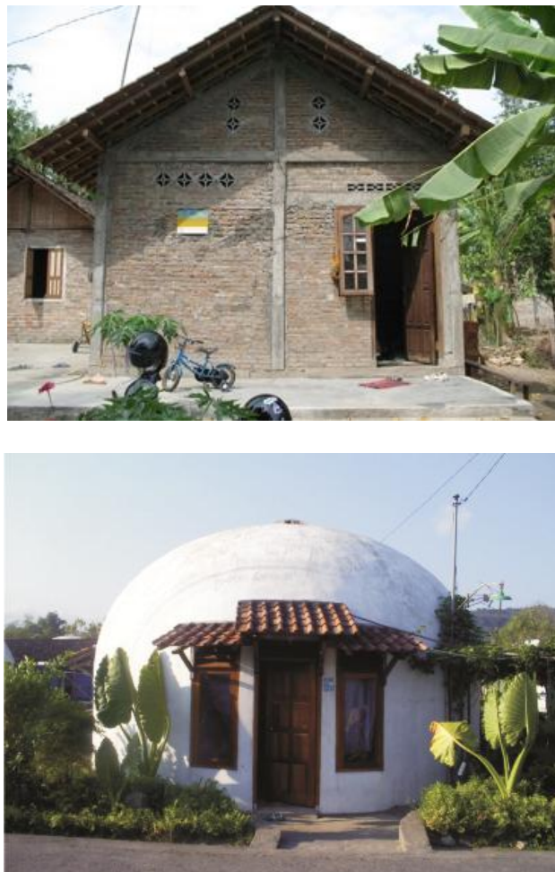
Figure 3-7: Reconstructed Houses: An ordinary - reinforced concrete frame structure and the unusual domed or shell-shaped structure
