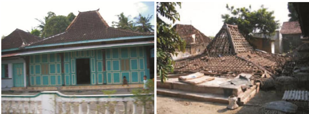
Figure 3-34: Traditional house with and without envelope wall after earthquake (right photo: Maer, B.W., 2008)
