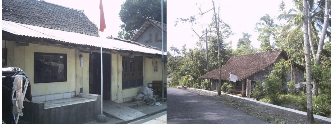
Figure 4-2: Similar Kampung type in Bantul before the earthquake (destroyed) and other area in Sleman after earthquake (undamaged)
