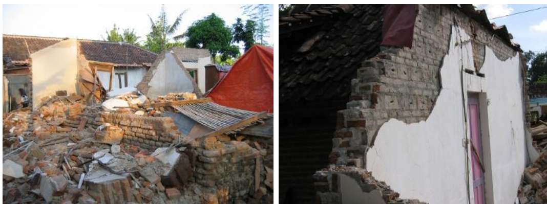
Figure 3-16: The most destroyed houses by weak unreinforced masonry wall (EERI 2006)
