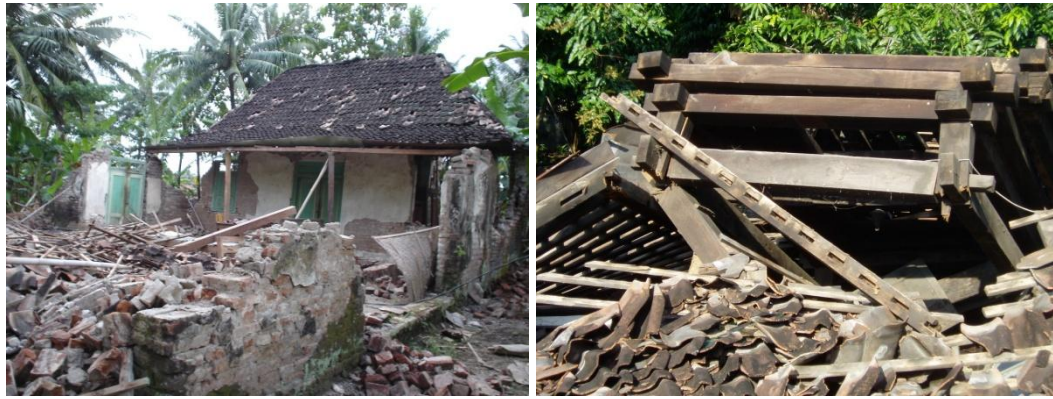
Figure 1-4 : Collapsed Houses; Brick wall bearing construction and wooden frame structure
