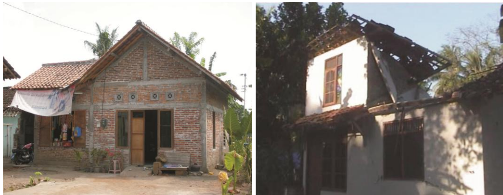
Figure 3-32: Missing column sample and the sample result from earthquake
