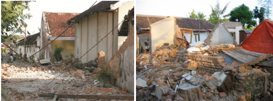
Figure 3-35: Masonry heavy wall failures
