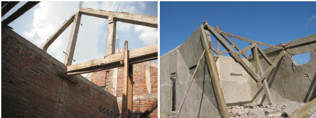
Figure 3-41: Heavy roof frame and its failure after earthquake (right photo: EERI, 2006)
