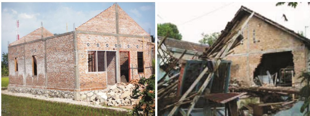
Figure 3-39: Incomplete frame for roof structure and its failure after earthquake (right photo: Boen, 2007)
