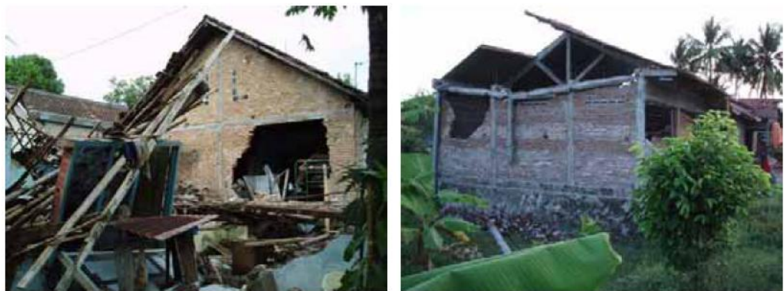
Figure 3-13: The destroyed masonry thin walled with RC frame (new culture) (Boen, 2006)
