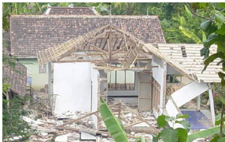
Figure 3-17: The destructed modern-vernacular type of Javanese Houses (Elnashai, A.S., et.al , 2007)
