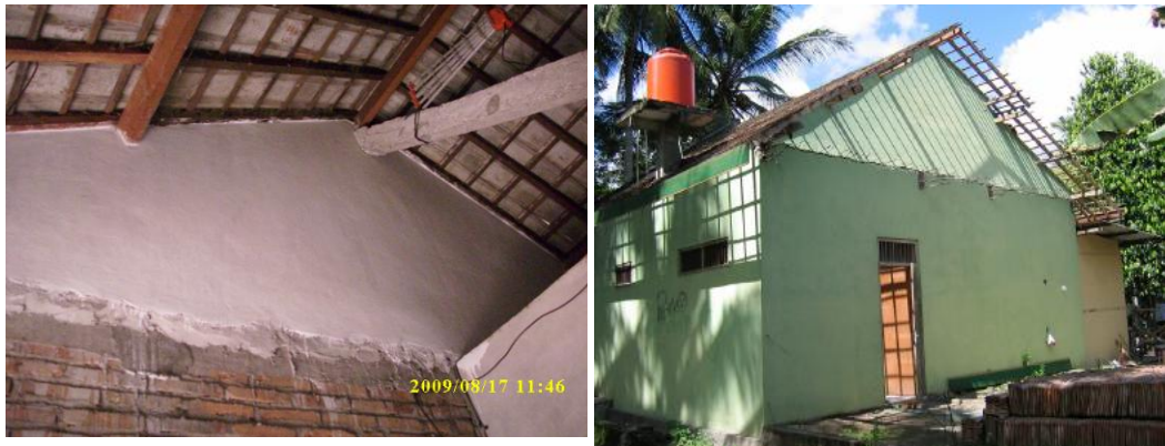
Figure 3-40: Supported-heavy roof frame and failure of unsupported framed or the absence of horizontal beam in between of gable roof (right photo: EERI, 2006)
