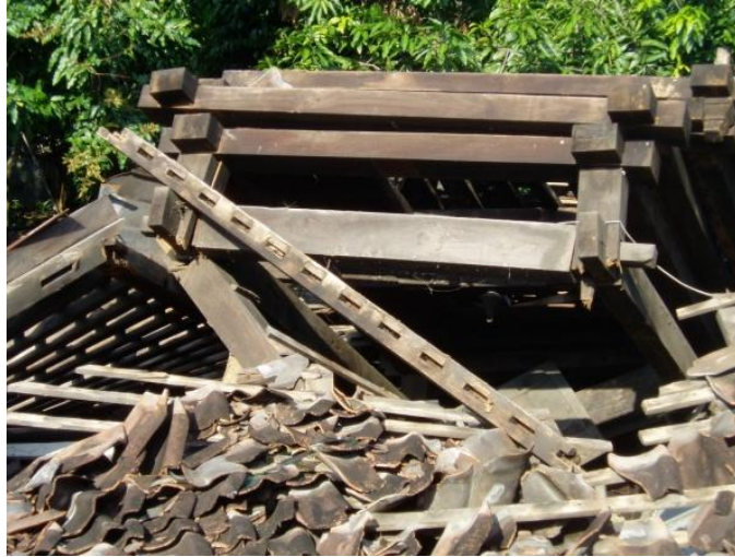
Figure 3-43: Connection failure of old and less maintained wooden structure
