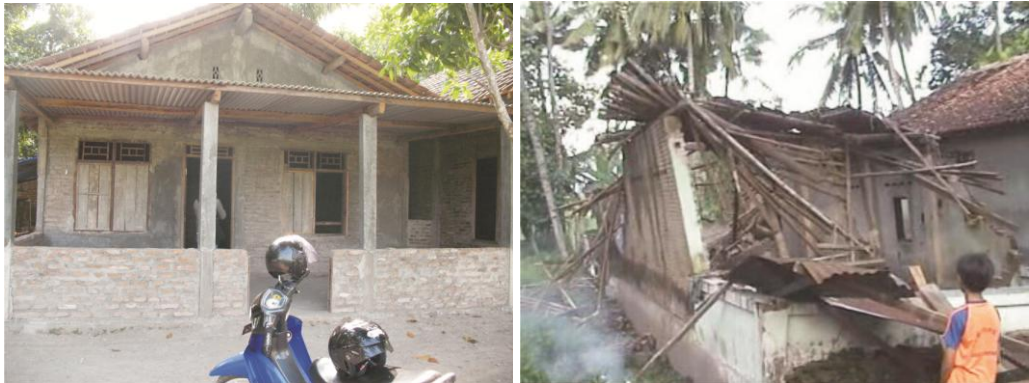
Figure 3-33: House sample without beam and the result from earthquake
