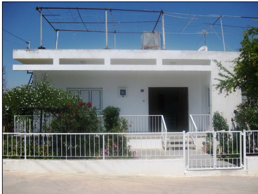
Figure 38 Modern rural dwelling, Çayırova village.
