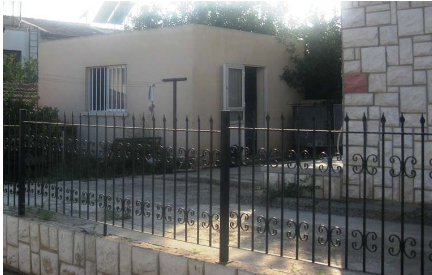
Figure 48 Secondary kitchen building.
