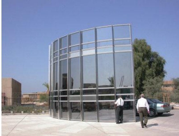
Picture 12: Tower Exterior Walls Brought to Site for Enveloping the Building (Peter. A. W, Gregory L. S, Mohamed. S, Skidmore, Owings & Merrill. 2007)
