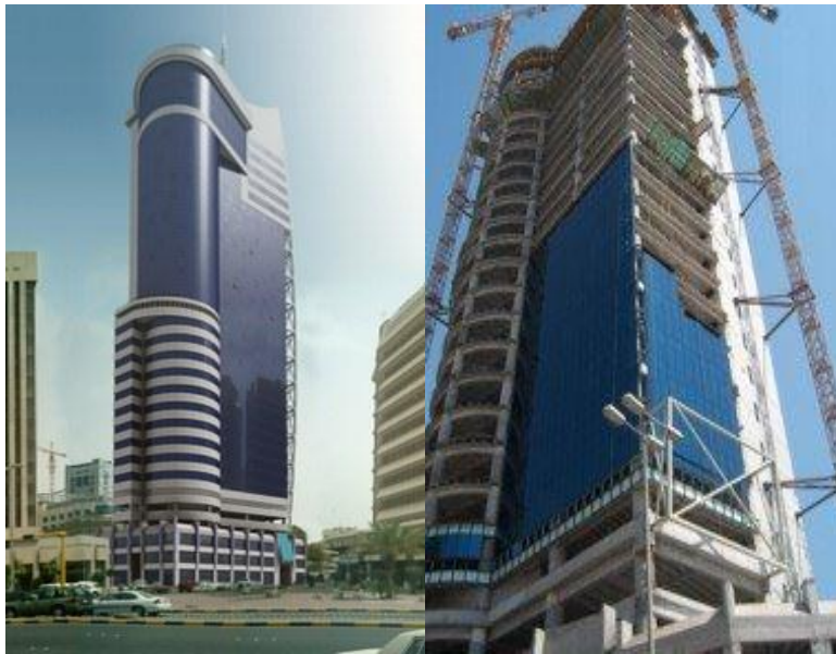
Picture 8: Al-Jawhara Tower with its Unitized Curtain Wall Installation Process (Futooh Al-Asfoor Consultant Engineers)
