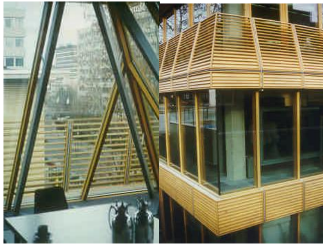
Picture 16: The Interior Part of the Curtain Wall Type and Image of Glazed Corner Detail (Fassaden Windows, 2009)
