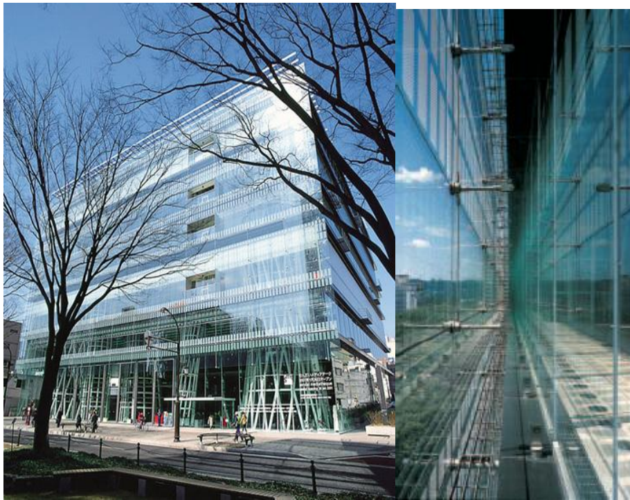
Picture 21: The South Facing Media Center Facade View and the Curtain Wall Connection (Schittich, C. 2001)
