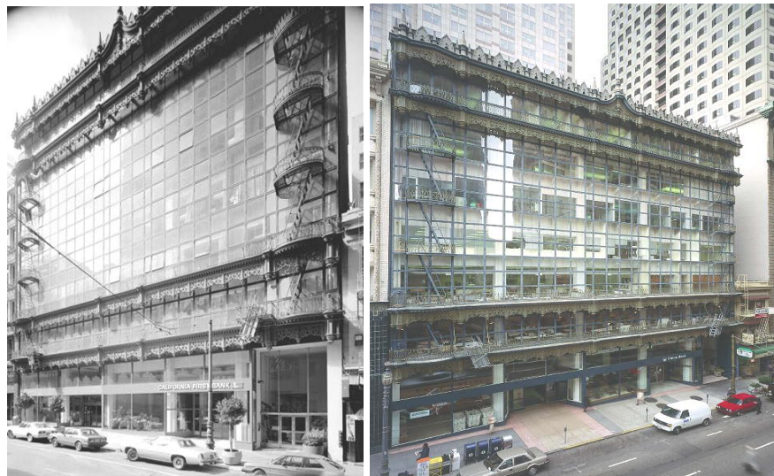
Picture 2: Hallidie Building in San Francisco Founded in 1918 by Willis Polk Curtain wall facade trimmed with cast iron detail.
