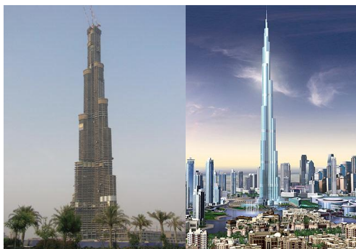
Picture 11: Panelized Curtain Wall System of Burj Tower, Dubai Architect/Structural Engineer/MEP Engineers: Skidmore, Owings & Merrill LLP. Year: 2004-2009
