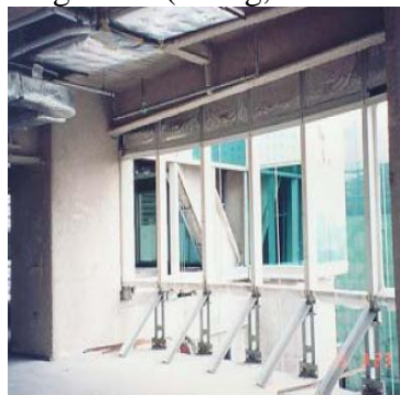
Picture 26: An Image of the Mullion and Transom Erection (Wong, W. M. R).
