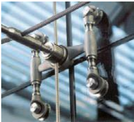
Picture 30: Sliding Spider Casting with Spring Loaded Arms Allows for High Seismic
