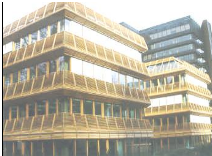
Picture 15: Office Building in Düsseldorf . Timber Spandrel Curtain Wall System. Year 1999. Germany Architects: Petzinka, Pink und Partner ( Fassaden Windows, 2009).
