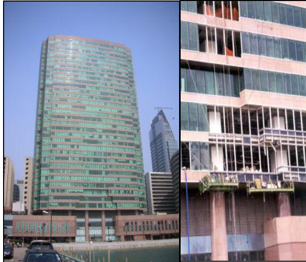
Picture 4: The Stick System of Gateway Tower 6 Commercial Building in TsimShaTsui Hong Kong. Architect: Wong and Ouyang (HK) Limited, Year built: 1991-1992 (Emphoris Corporation. 2000-2009).
