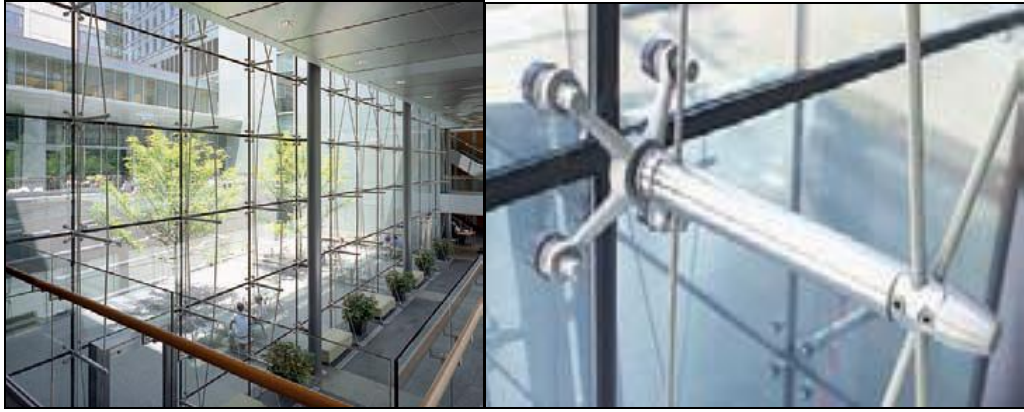
Picture 31: Harvard Medical School – New Research Building. Stainless Steel Nexus Castings and Articulated 902 Boston, MA. Architect: Architectural Resources Cambridge, Inc (Pilkington Planar Catalog. 2007)
