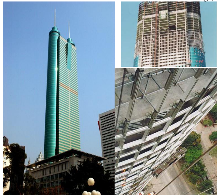
Picture 6: Shun Hing Plaza Stick Curtain Wall System. Year built: 1993-1996 Architect: K.Y. Cheung Design Associates. http://en.wikipedia.org/wiki/Shun_Hing_Square
