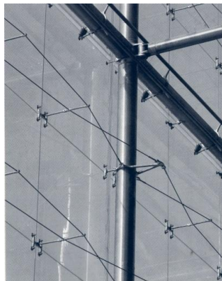
Picture 24: Typical Stainless Steel Profile (structural steel frame) for Curtain Wall System (Peter and Dutton, 1995)
