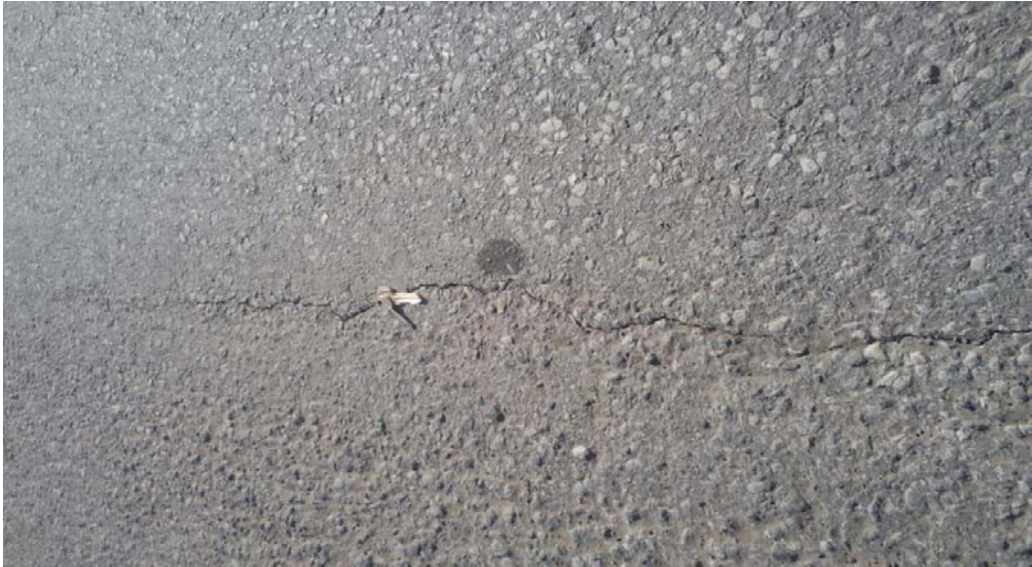
Figure 56: Transverse, Low Severity
