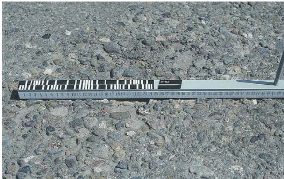
Figure 20: Loss of Coarse Aggregate (Miller, J. S., & Bellinger, W. Y., 2003, p. 28)
