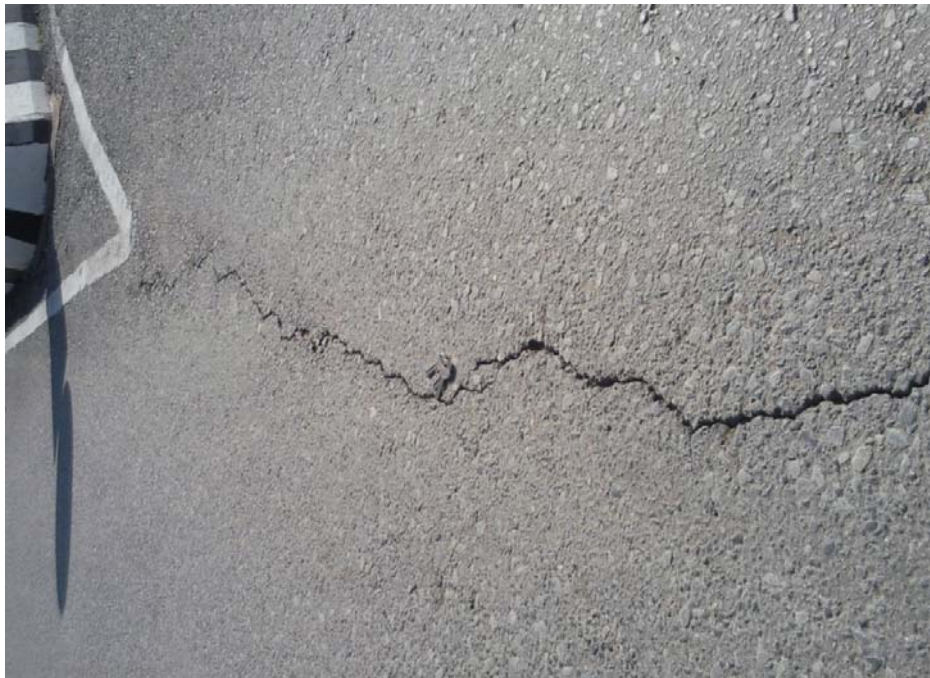
Figure 54: Transverse, High Severity
