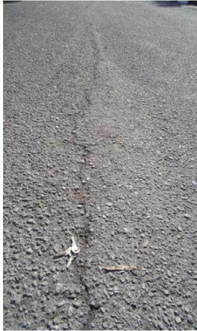
Figure 53: Longitudinal, Low Severity
