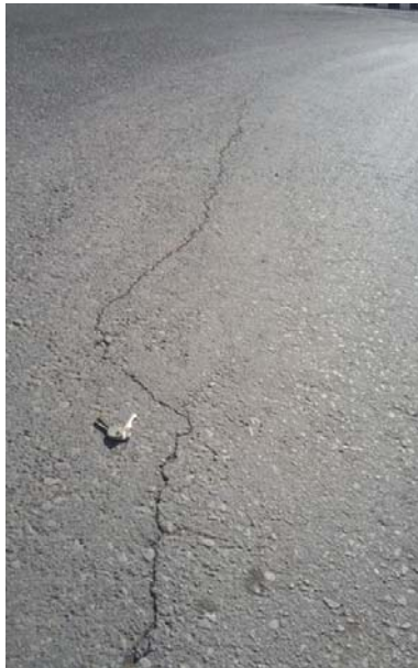
Figure 52: Longitudinal, Medium Severity
