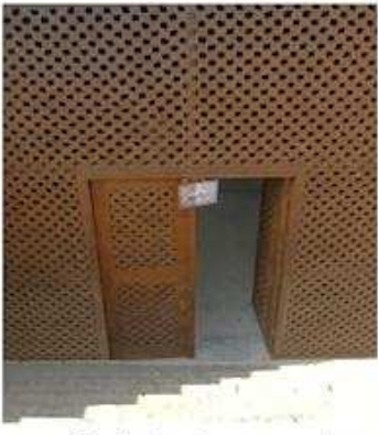
Stair to basement
