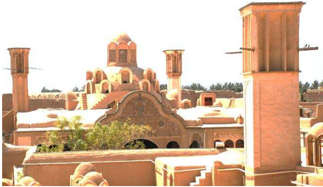
Figure 53. View of arched roof of Kashan house. Photo by Hamzeh Karbasi.
