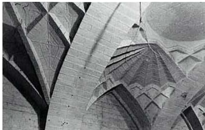
Figure 53: Ceilings in ‘Neem Sardab’ in traditional Baghdad house (Warren & Fethi 1982)
