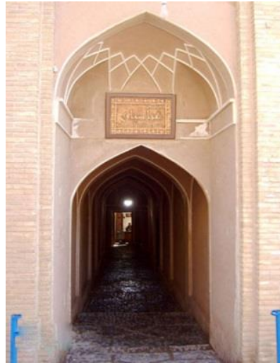
Figure 5: Dalan of Abbasi house in kashan (taken by author, 2012)
