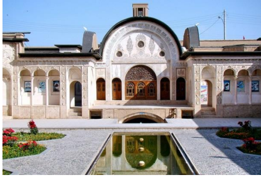
Figure 65: Major Courtyard in Tabatabaee House (taken by author, 2012)
