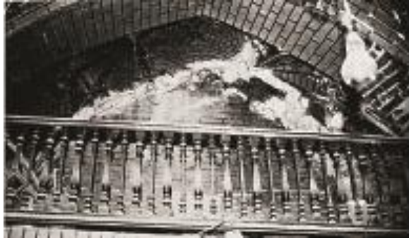
Figure 51: 'Takhta-Boosh' in Baghdad traditional house (Warren & Fethi 1982)
