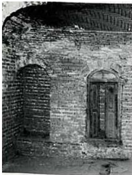
Figure 50: 'Badgir' opening in a 'Neem sardab' in Baghdad traditional house (Warren & Fethi 1982)
