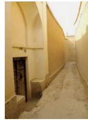
Traditional Facade in Kashan
