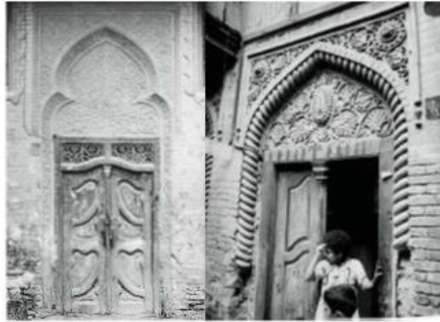
Figure 32: wooden entrance door in Baghdad traditional house (Warren & Fethi, 1982)
