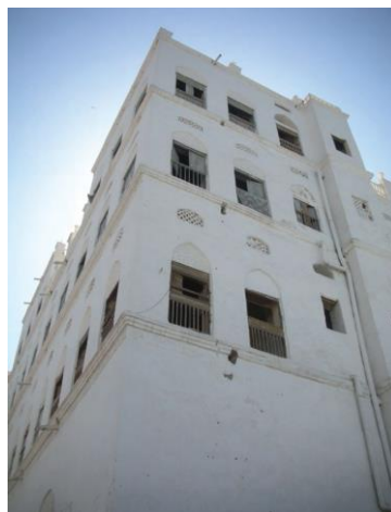
Figure 22: Mukalla windows of house (Baeissa, 2011)
