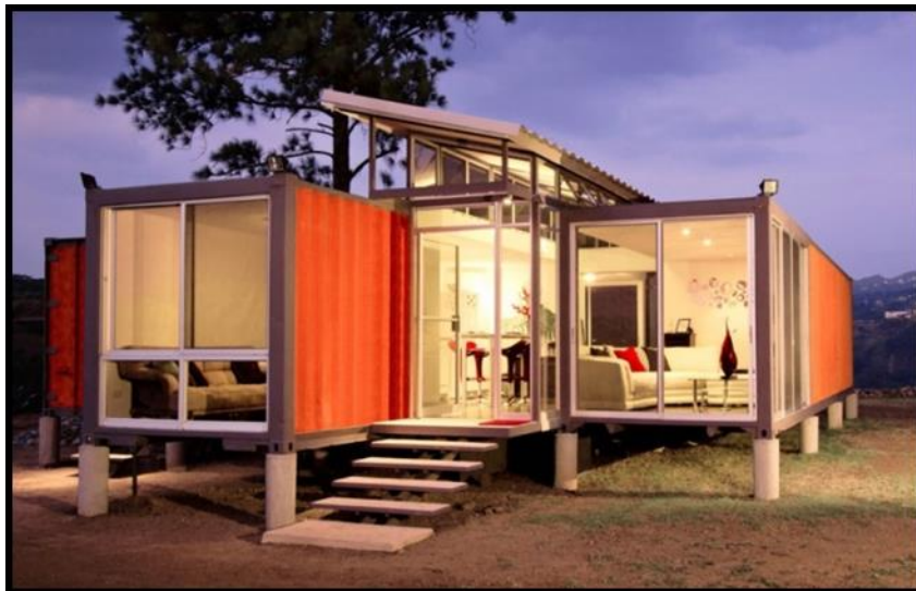
Figure 31: Exterior View of a Container House (Homedsn, 2011)
