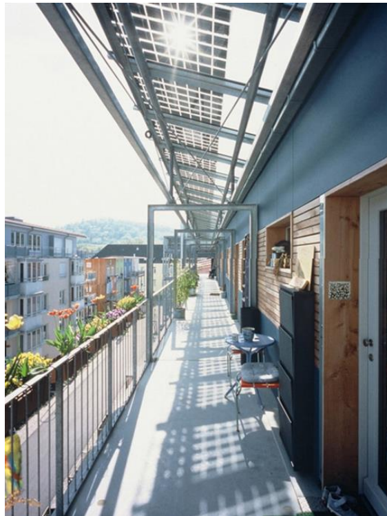
Figure 61: Access balcony with photovoltaics inclined southwards (Voss et al., 2013)
