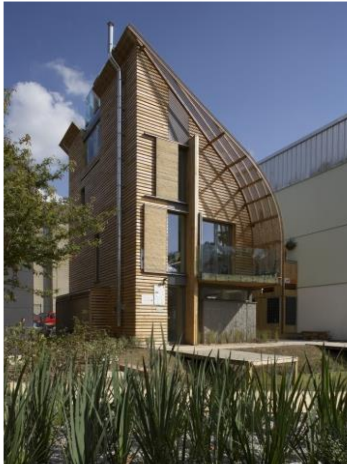
Figure 49: Building view of light house (Kingspan, 2007)
