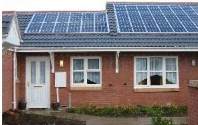
Figure 13: Photovoltaic Roof System (Sharma, 2014)
