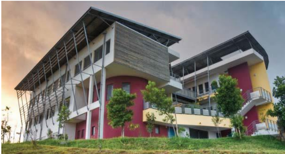
Figure 64: Building view of University building, LA Reunion Island (Voss et al., 2013)
