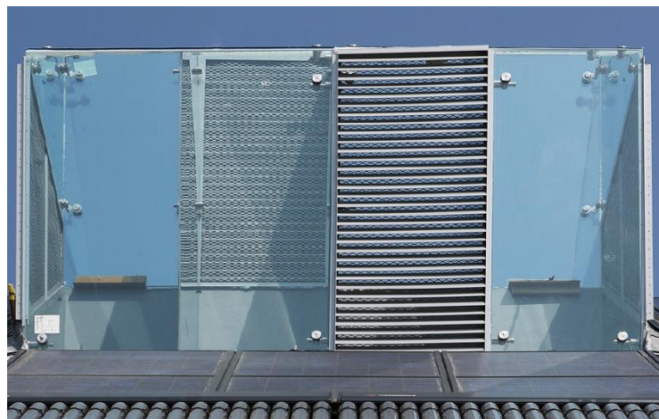
Figure 54: Wind catcher (Kingspan, 2007)
