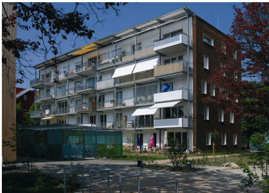
Figure 62: South- East view of Klee House (Voss et al., 2013)
