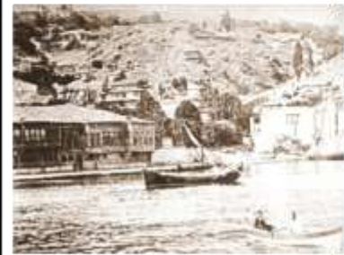
A view of the historic mansion before conservation
