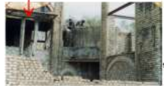
Rooms under construction
