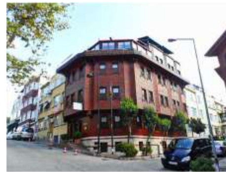
A view of Dersaadet hotel after conservation
