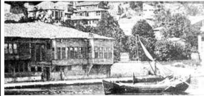
A view of the historic mansion before conservation
