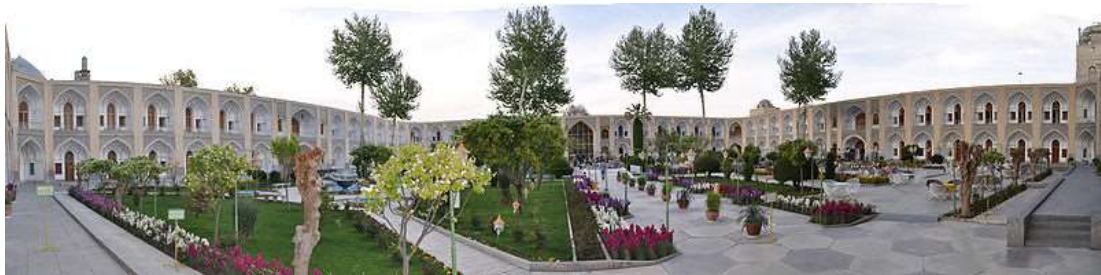
Figure 16. Abbasi Hotel. Isfahan, Iran (Abbasi Hotel)
