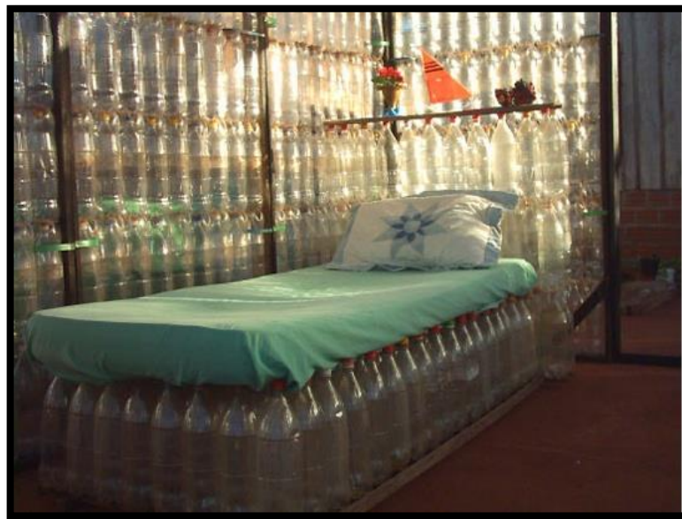
Figure 27. A bed and interior wall made by recycled materials by using recycle plastic instead of trashing them. (Inhabitots, 2010)
