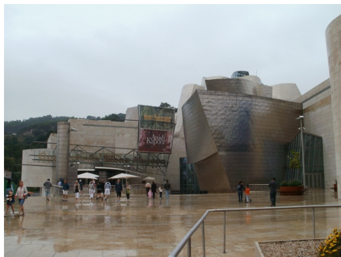
Figure 32: Guggenheim museum Bilbao (Source: Personal Archive)
