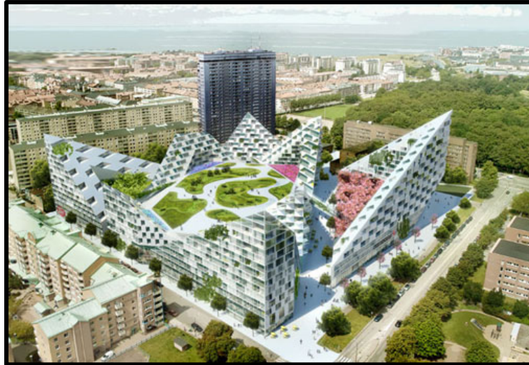
Figure 7. Open space in architecture (URL4)
