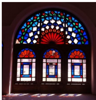
Figure 46: Sash Window (Orosi), “Tabatabai Residence”, Kashan, IRAN (Photograph by Author)
