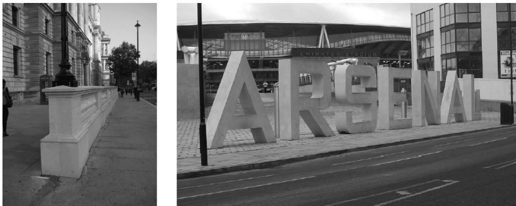
Figure 2. Left: Security Balustrade along Whitehall, London. Right: ARSENAL, Ornamental security facade for the Emirates Stadium (Coaffee, O'hare, & Hawkesworth, 2009).
