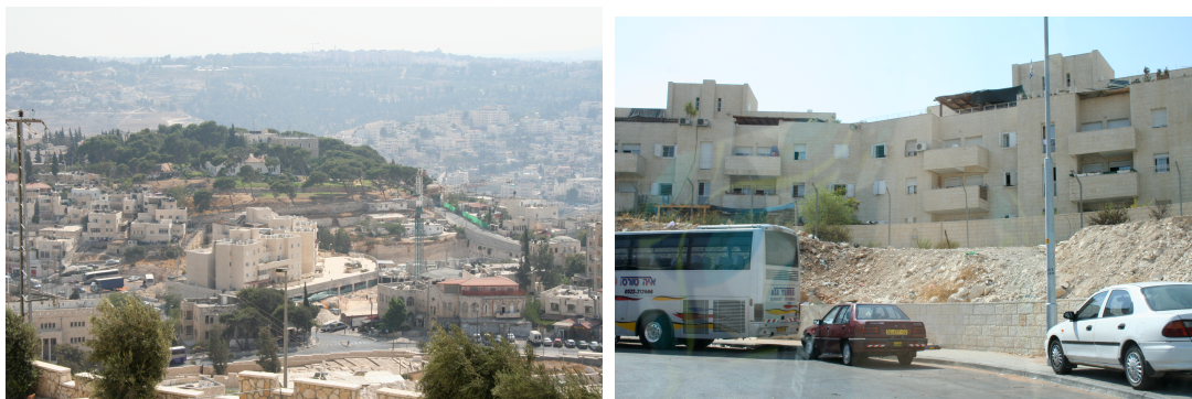
Figure 29. The elevated Israeli building block on Ras el Amood hilltop (Photo: Author, 2008).
