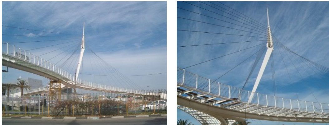
Figure 44. The bridge designed by Santiago Calatrava in Petik Tikva, near Tel-Aviv (URL 3, 2006).
