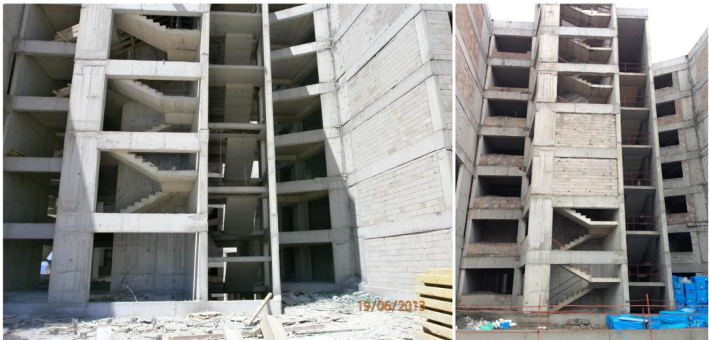
Figure 5.7. Guardrails in staircases (3)
