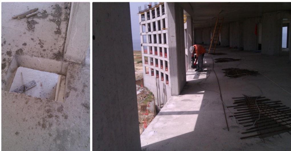
Figure 5.12. Floor covers for openings
