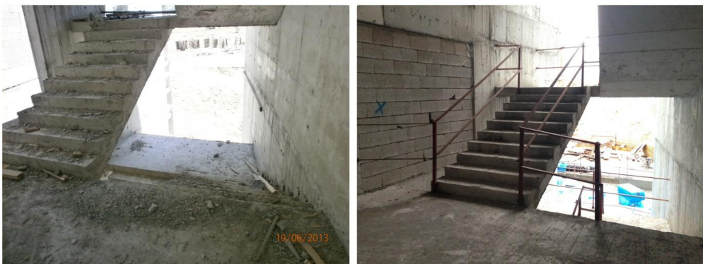
Figure 5.6. Guardrails in staircases (2)
