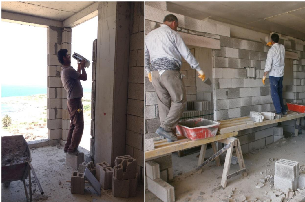
Figure 5.13. Work at height level
