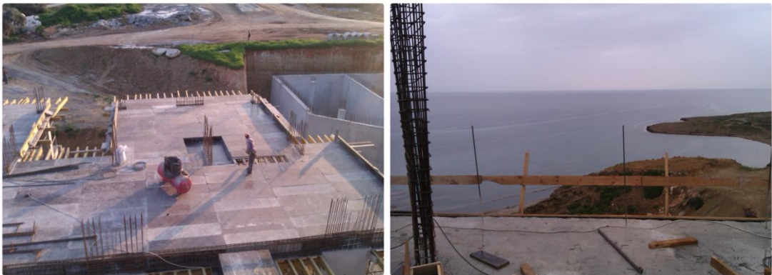
Figure 5.4. Guardrails in LPH project
