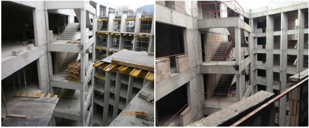
Figure 5.5 Guardrails in staircases (1)
