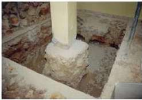
(a) Excavating around the footing
