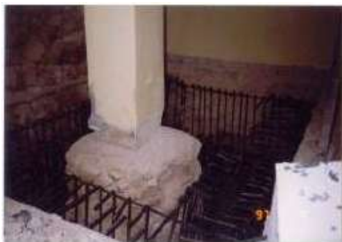
(c) Installing the main steel
