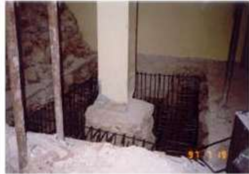
(b) Hardening the surface and installing the dowels
