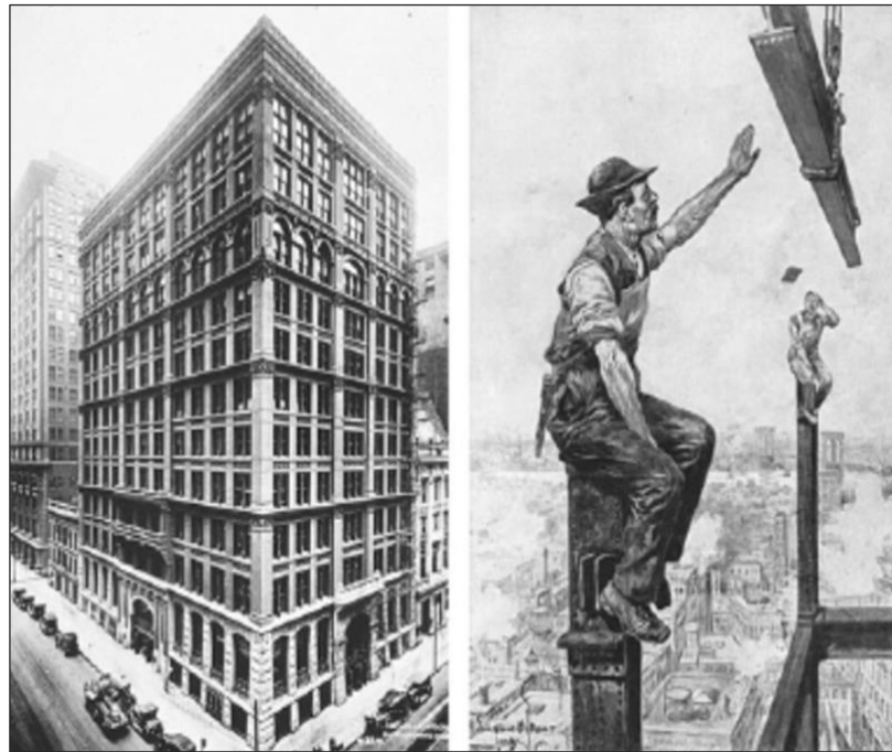
Figure 2.4: The first skyscraper with load-carrying frame of steel structure, Source: (Vaclav, 2005)
