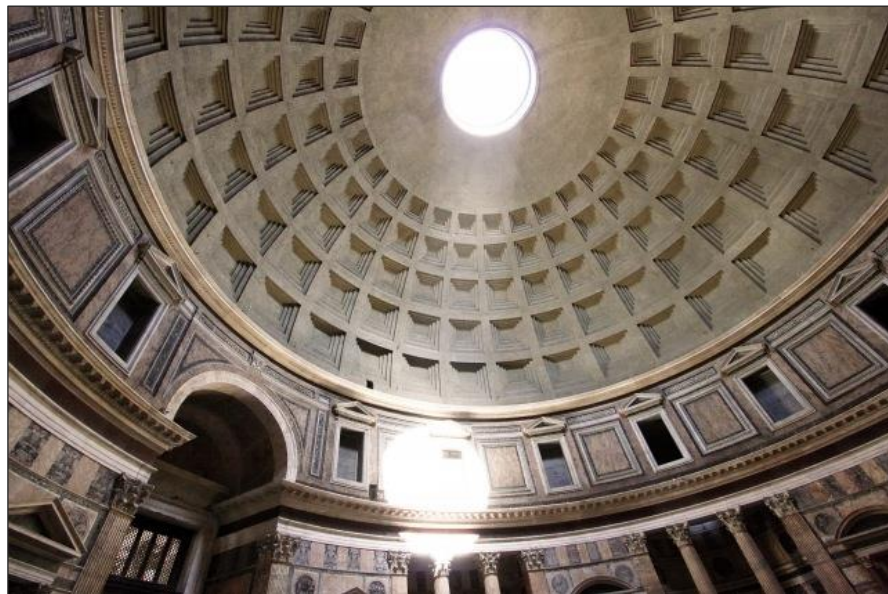
Figure 2.2: Inside the Pantheon (2nd c.); on the lowest level travertine, the then a mixture of travertine and tufa, then tufa and brick, then all brick was used around the drum section of dome, and finally pumice as the lightest and porous materials for the ceiling of dome. Source: (URL2; URL3)
