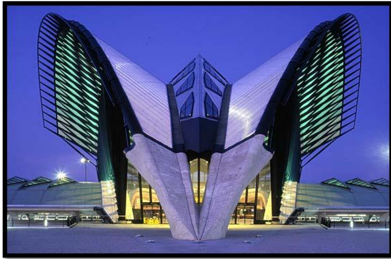
Figure 25. The Building's Most Striking Profile; Showing the Two Converging Steel Arches With Expressive of a Bird, Symbolizing Flight. (URL17)
