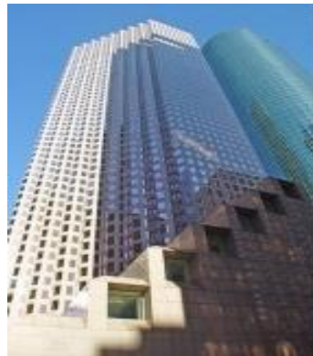
Figure 34. Contrast between old and new parts of building (URL 25)
