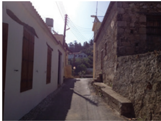
Figure 2. Current situation of Beylerbeyi Olive oil Mills (First one is on the right side; Second one is on the left side) (Eken and Varol, 2014)
