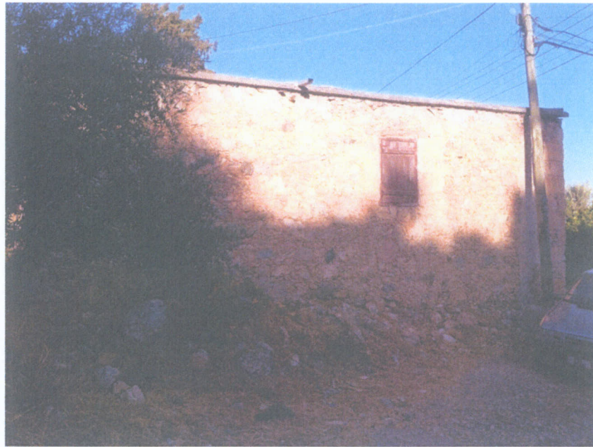
Figure 30. Example from traditional Aghirda (Ağırdağ) houses constructed with stone masonry (Author, 2012)
