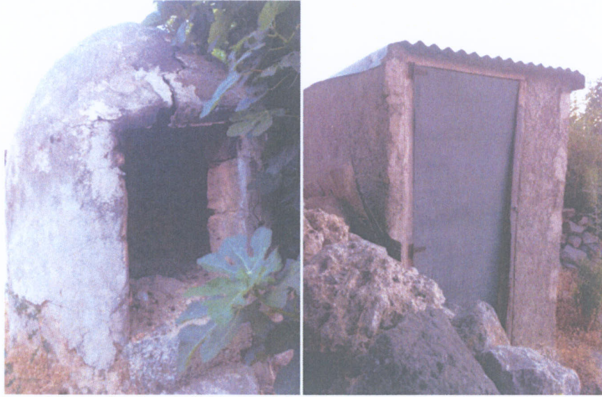
Figure 11.Examples from toilet in Aghirda (Ağırdağ) traditional houses (Author,2012)
