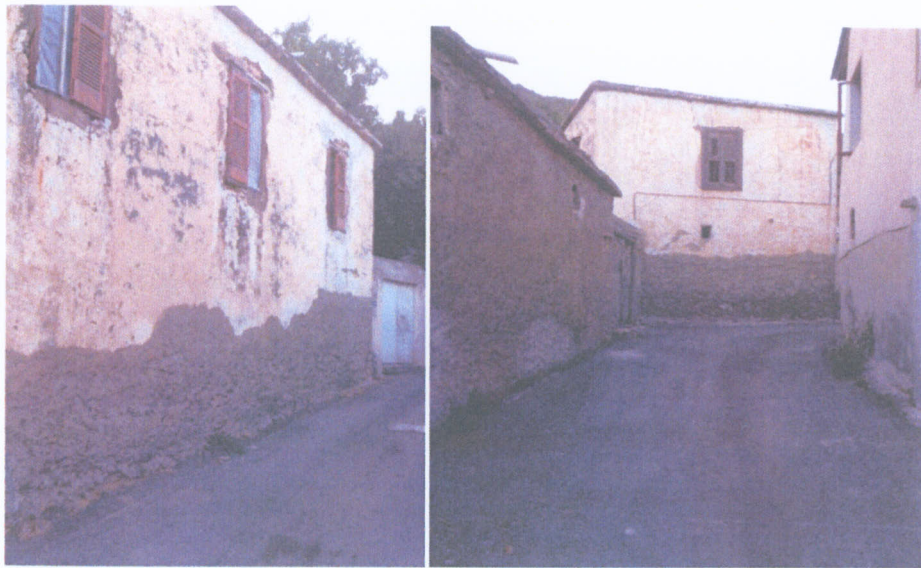
Figure 31. Examples from mud construction material and whitewashed wall surfaces (Author,2012)
