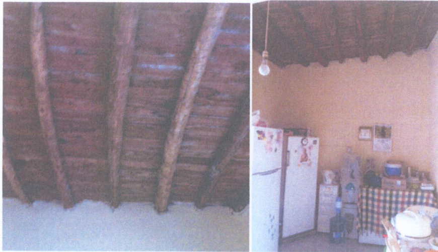
Figure 32.Examples from wooden beams on the roof structure of traditional Aghirda (Ağırdağ) houses (Author,2012)
