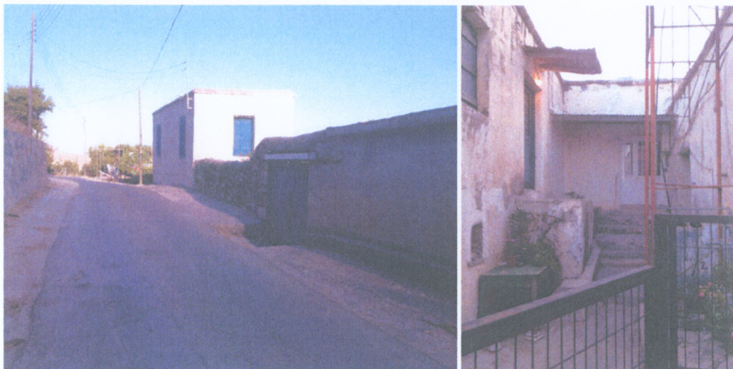
Figure 18.Examples from street- yard-house relations of analyzed houses (Author,2012)
