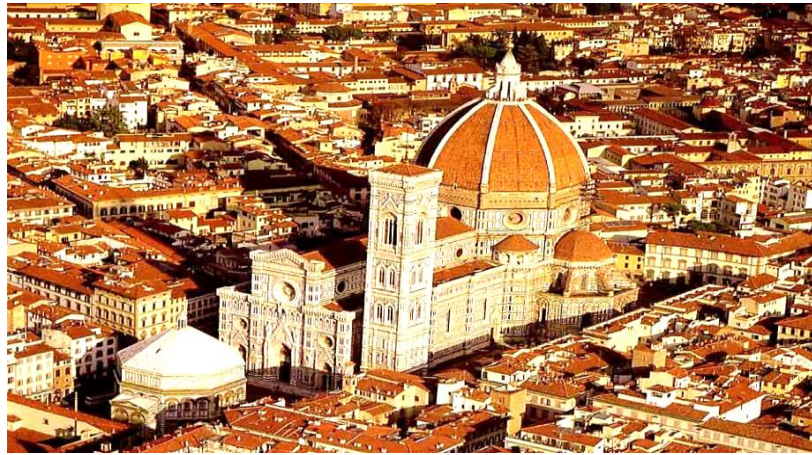
Figure 4.16. The cathedral of Santa Maria del Fiore in Florence Source: http://www.arch.mcgill.com
