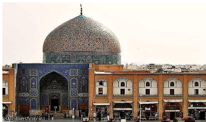
Figure 4.36. Sheikh Lotfallah Mosque Source: http://www.shabestan.ir
