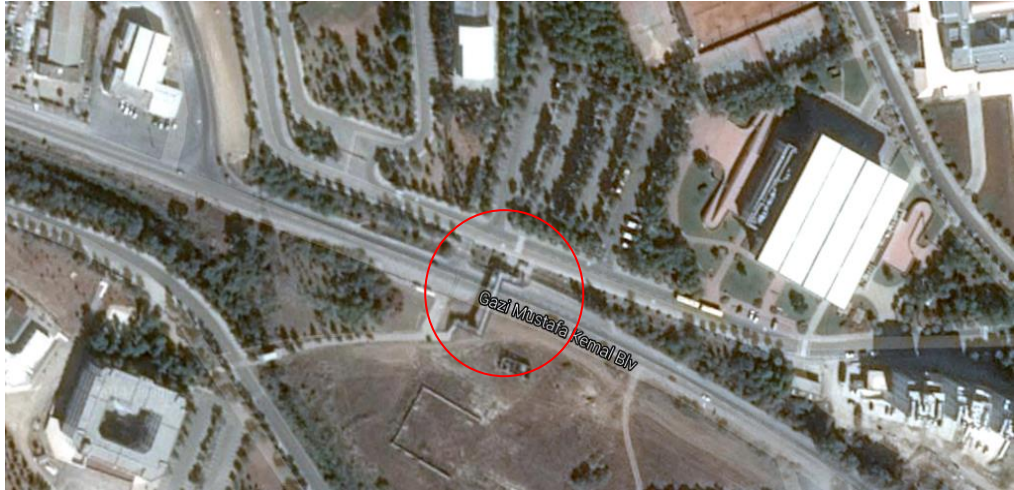
Figure 3.1: Satellite view of the bridge (obtained from Google map)
