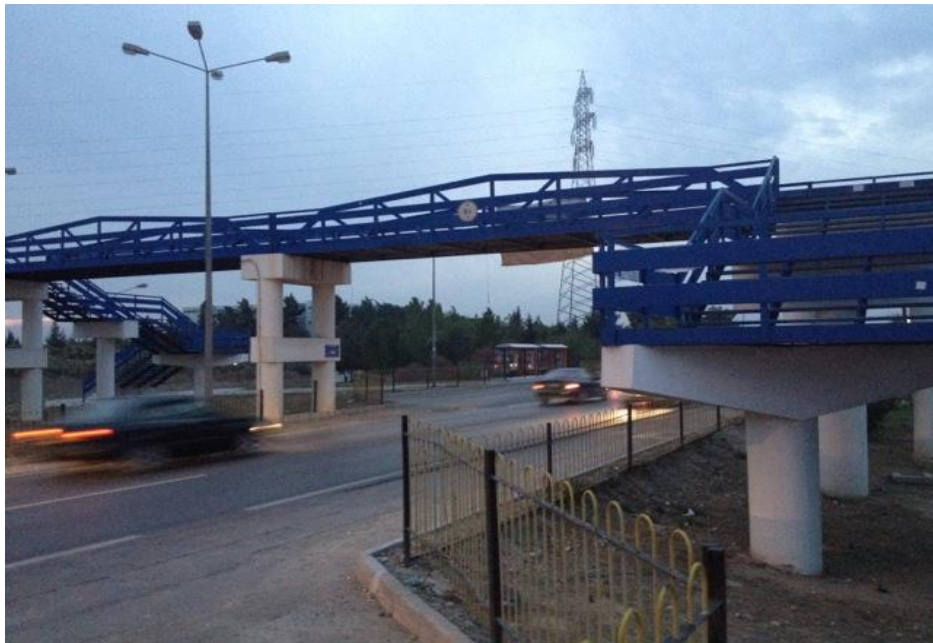
Figure 3.2: The photo of the constructed bridge
