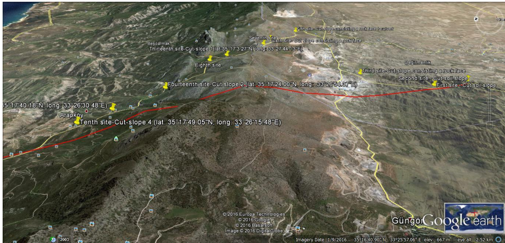
Figure A.2. Geotechnical assets along Kyrenia mountains range (with the courtesy of Google Earth ©).
