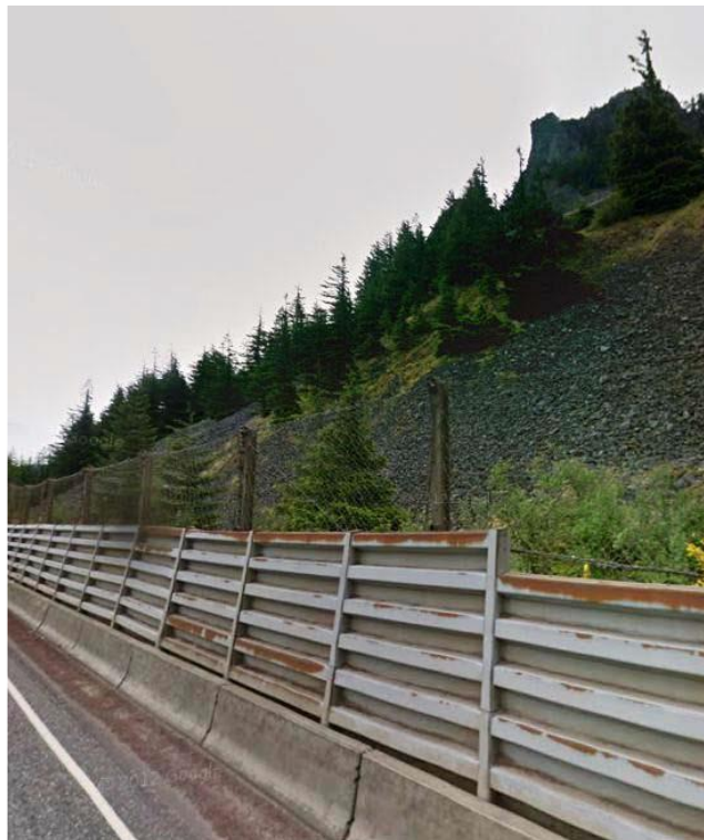
Figure 3.10. Net fence barrier (Fred Gullixson, & Peltz, 2013).
