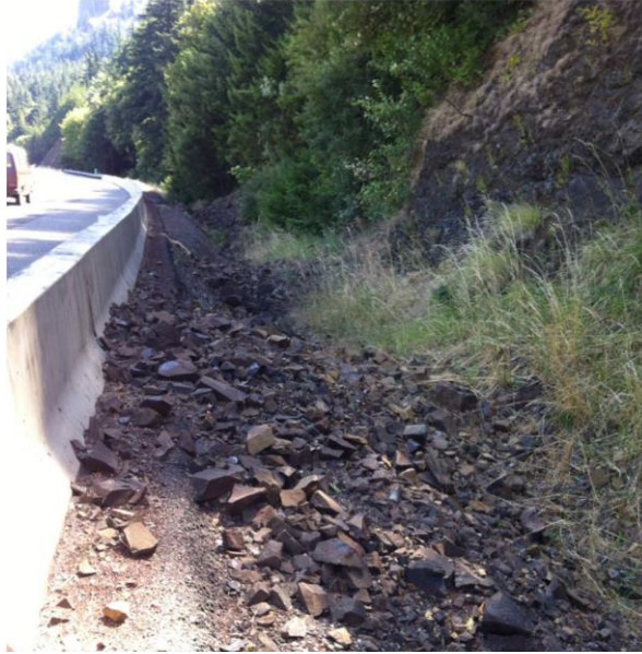
Figure 3.9. Rigid barrier (Fred Gullixson, & Peltz, 2013).
