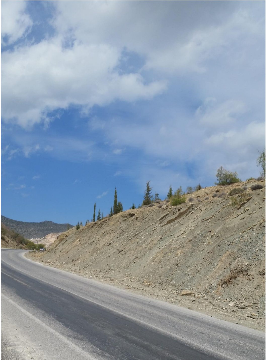
Figure D.6. Site 2-Eastern.
