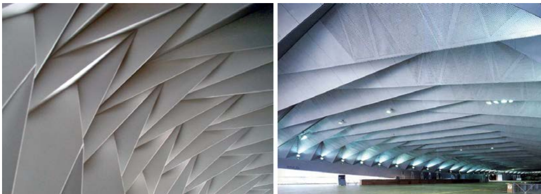
Figure 12: Paper folded model (left) and roof structure (right) of the Yokohama terminal by Foreign Office Architects.
