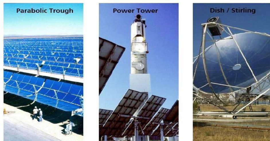
Figure 2.1. Solar Power Plants [15]
