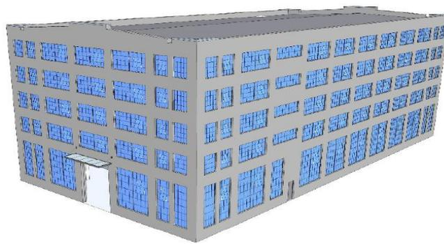
Figure 4.7. Illustration of a building with a soft ground story due to tall piers.
