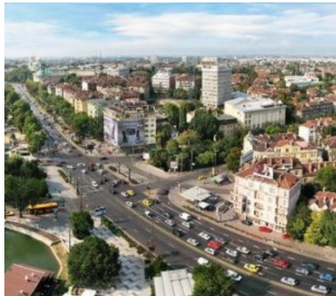
Figure 2.16. Arterial Street, USA (URL4)
