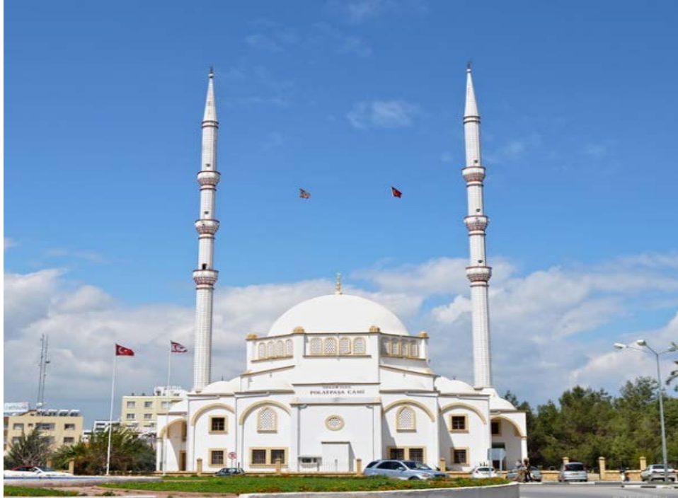
Figure 3.11. Osman Fazil Polat Pasha Mosque: Landmark in the city
