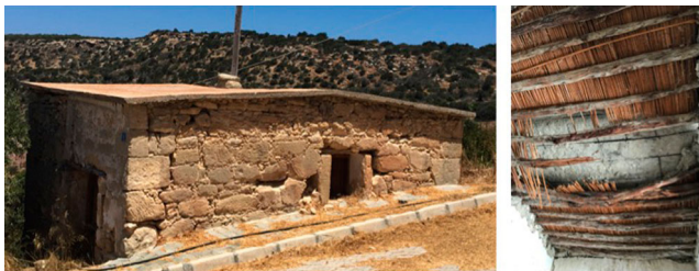
Figure 11. Concrete roof over Esenköy and Büyükkonuk 1 olive mills.
