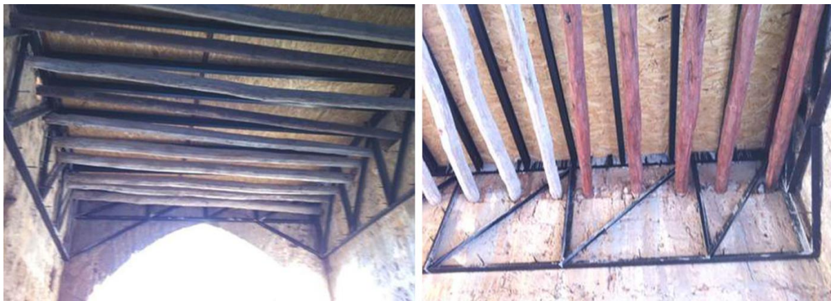
Fig. 8. Steel beams added during restoration work. (Photos by .....)
