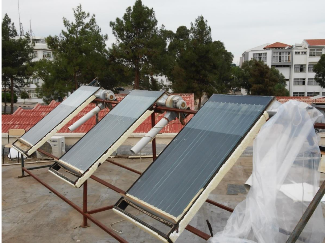
Figure 3. 2:Pictorial view of the experimental setup of three slit glazed solar air heaters.
