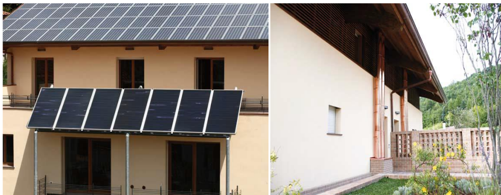
Figure 64 : photovoltaic (PV) integrated roof and use of roof as shading devices (URL 23).
