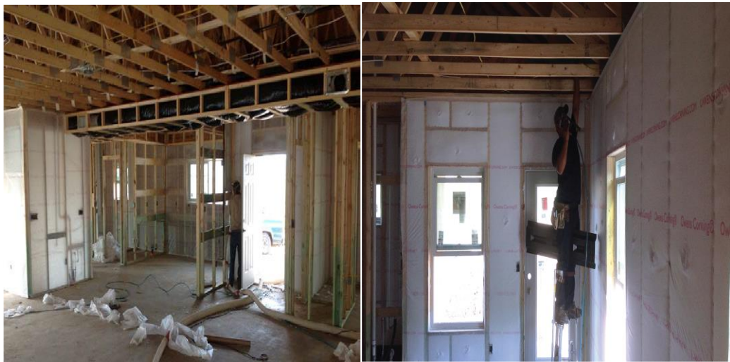
Figure 67 : show construction process and installing equipment (URL 1).
