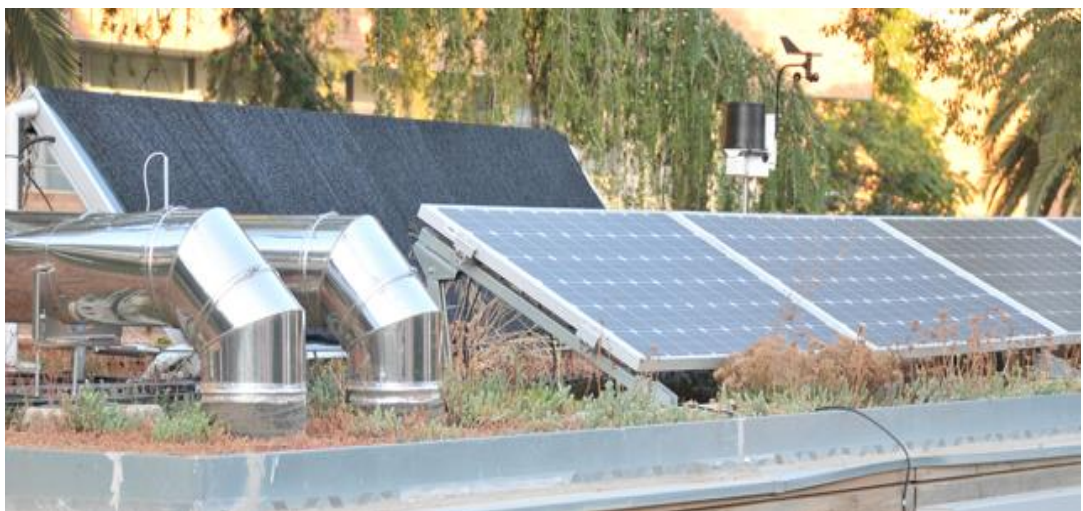
Figure 56 : roof of Lima house (URL 8).
