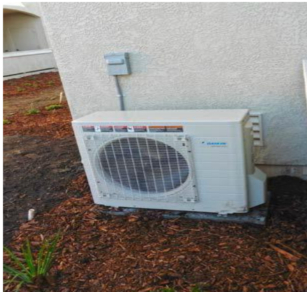
Figure 70 : The air-to-water heat pumps provide efficient, combustion-free heating, cooling, and hot water (URL 10).
