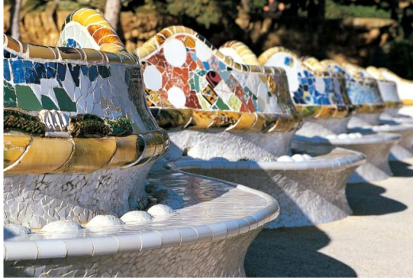
Figure 34: Picture shows repaired vandalism on tiles at Park Güell in 2007 (URL 3.14)
