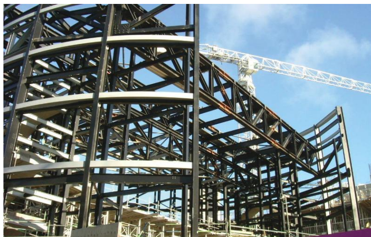
Figure 1.3: Ordinary truss moment frames (TMF) [3]
